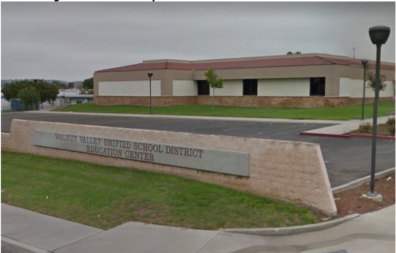
Figure 1: Walnut Valley Unified School District Education Center
