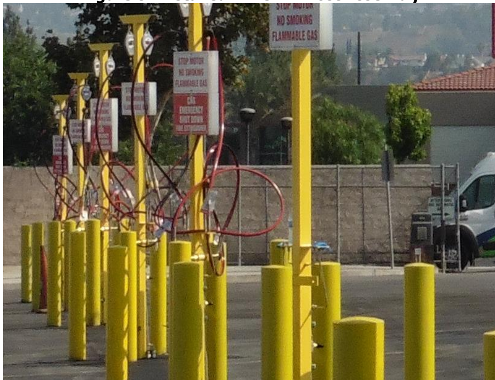
Figure 8: Installed Time-Fill Post Assembly
