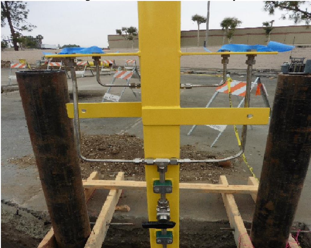
Figure 7: Time-Fill Post Assembly
