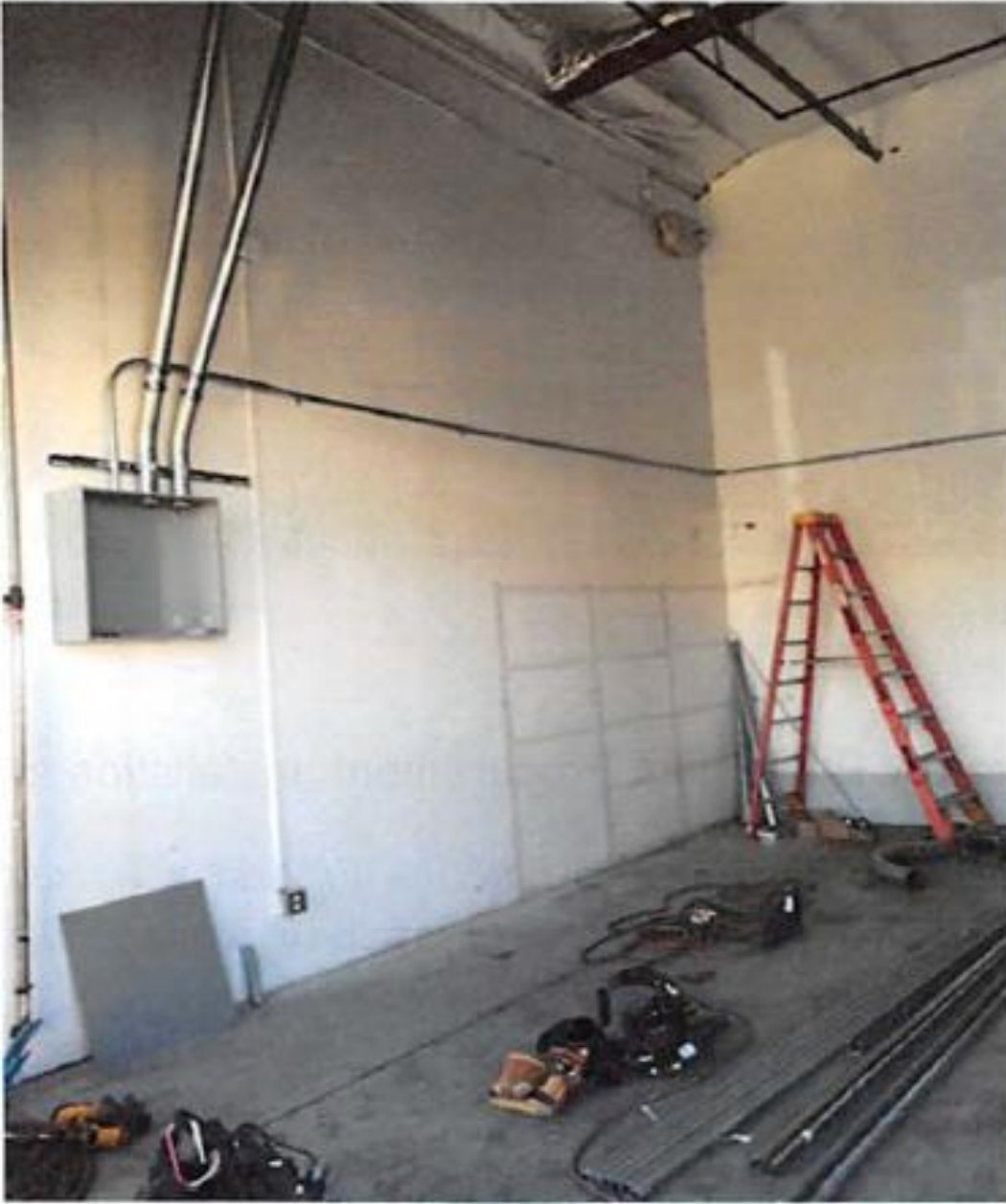
Figure 2: BMS Electronics Lab Electrical Work in Progress
