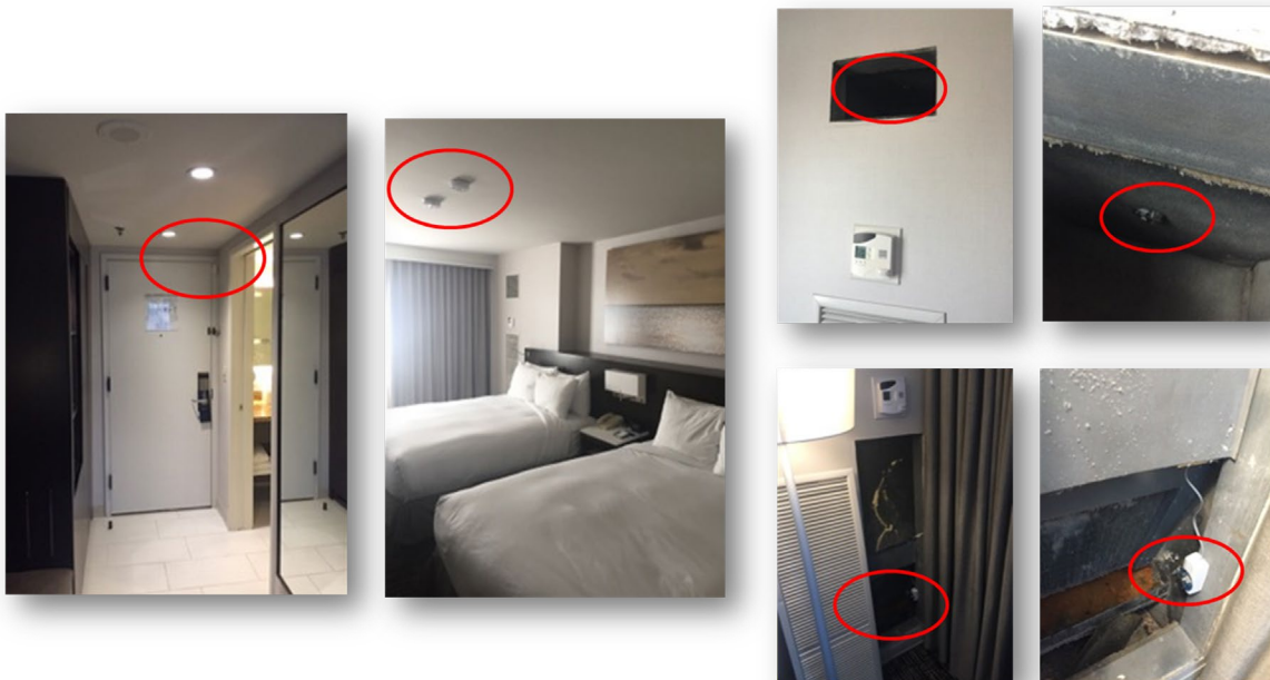
Figure 17: Guest Room Placement of Conectric Networks Sensors
