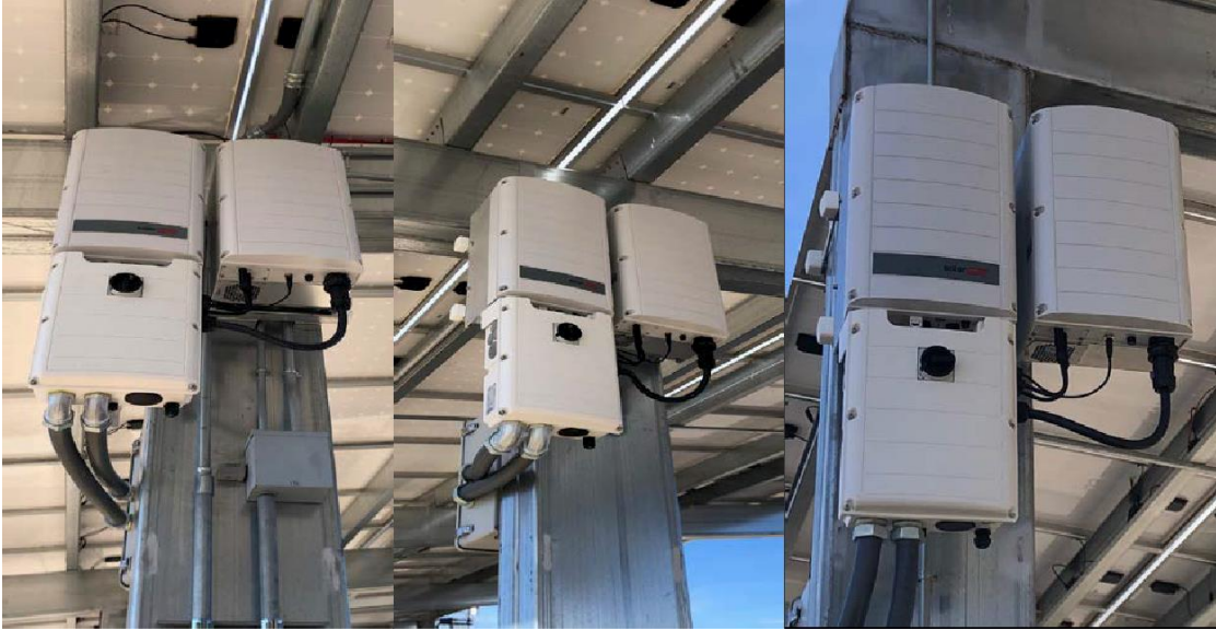
Figure 30: SolarEdge Inverter Installation
