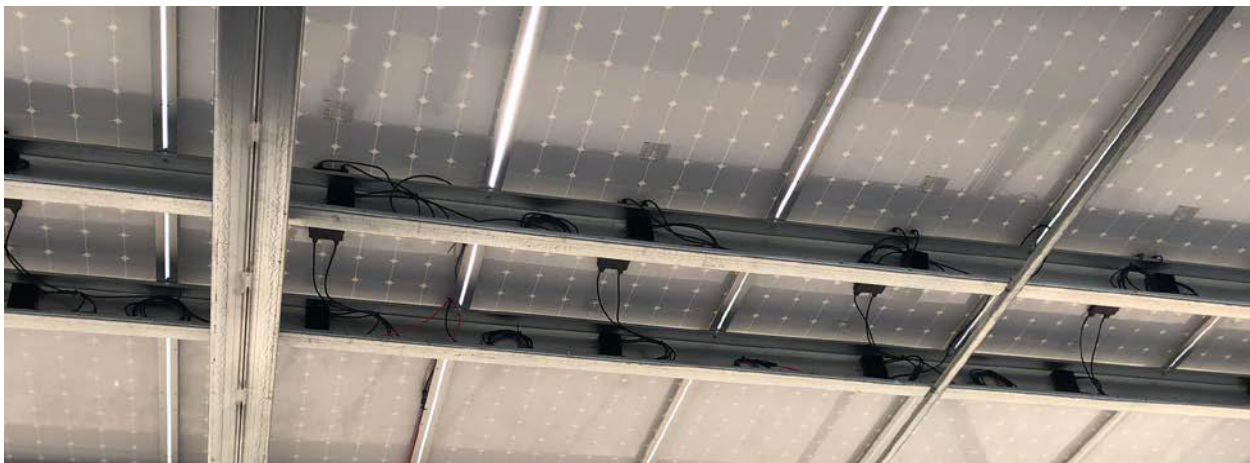
Figure 29: SolarEdge Optimizer Installation
