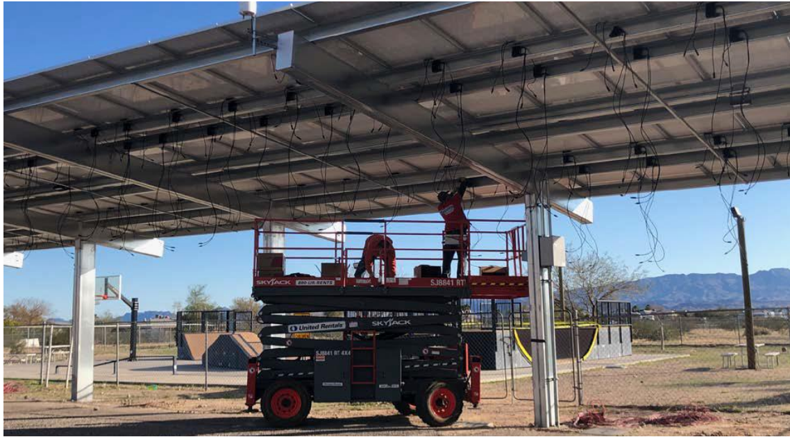
Figure 28: Solar Photovoltaic String Reconfiguration
