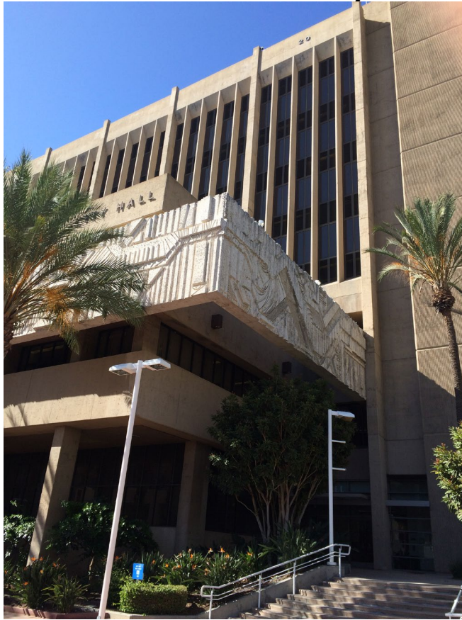
Figure 3: Exterior View of Santa Ana City Hall Office Tower
