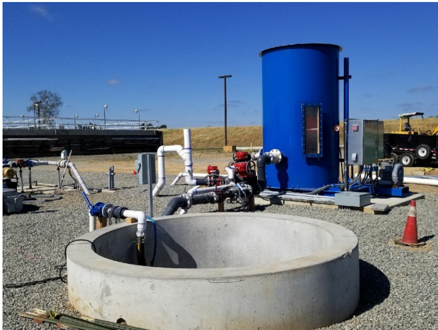
Newly Constructed Storage Vault No. 4.
