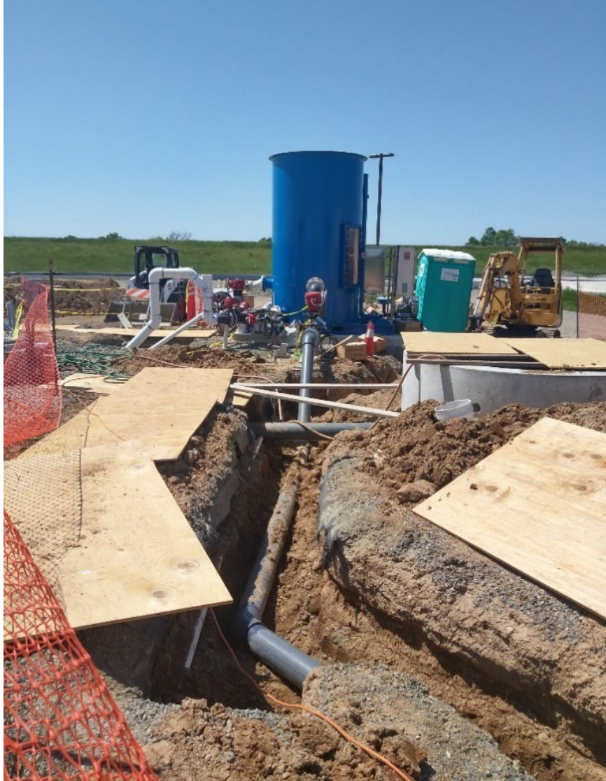
Construction of Biofiltration Demonstration System.
