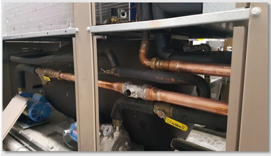
Figure 22: NIST-Calibrated Flow Meter Installed in Tube
