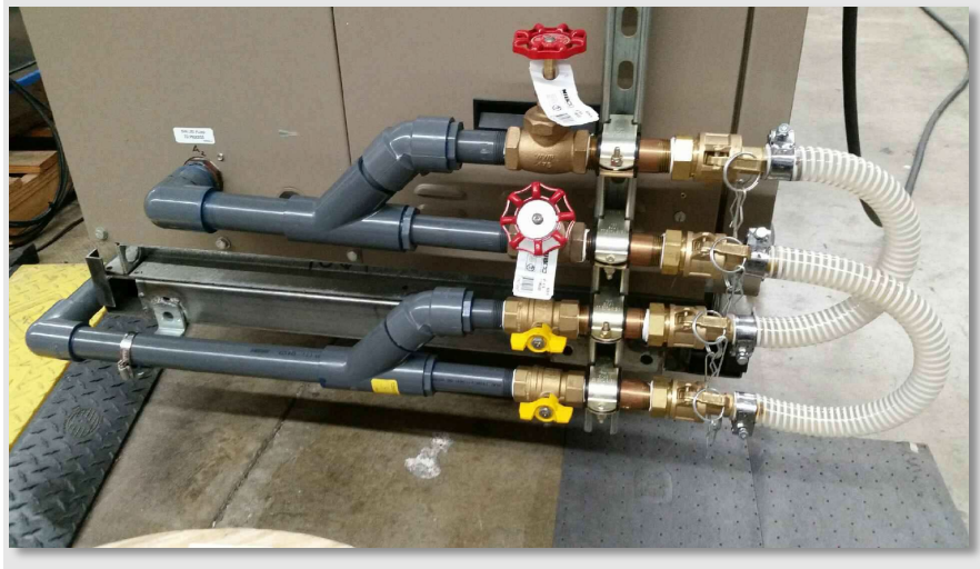
Figure 23: Chilled Process Water Connections for Fan-Coil Units
