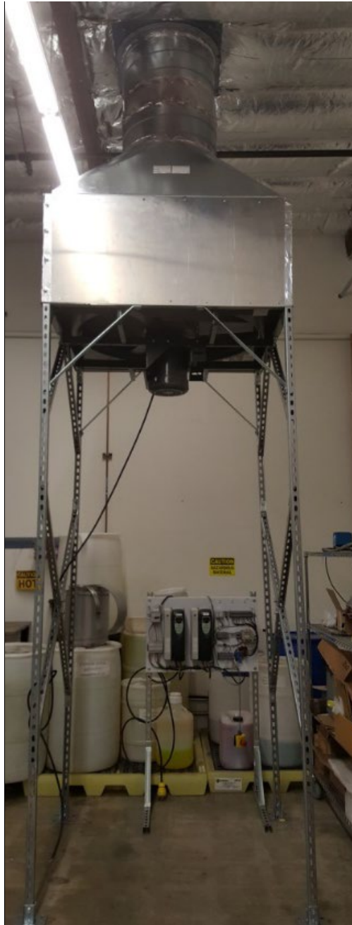
Figure 21: Condenser Hot Air Exhaust Duct Installation at Altex Facility
