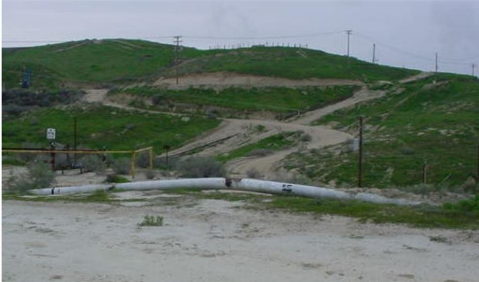
**An example of upheaval and buckling of gas pipelines resulting from subsidence caused by fluid extraction**
