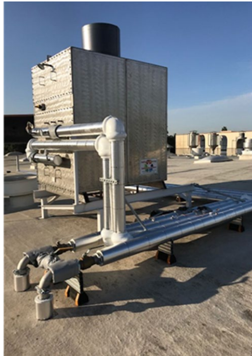
Figure 11: Installation of Economizer
