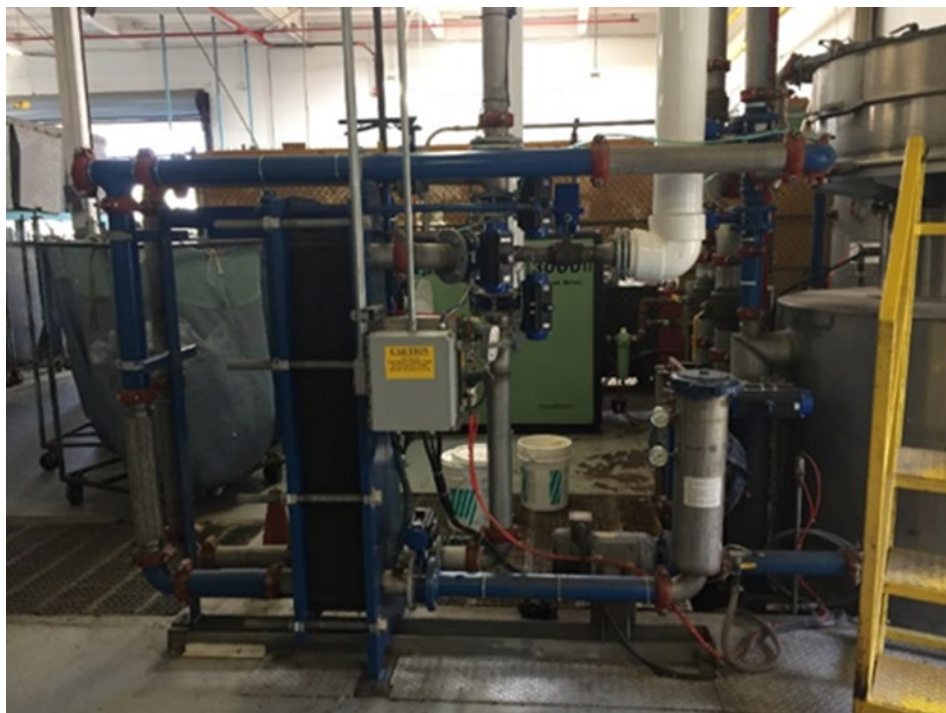
Figure 6: Wastewater Heat Recovery System
