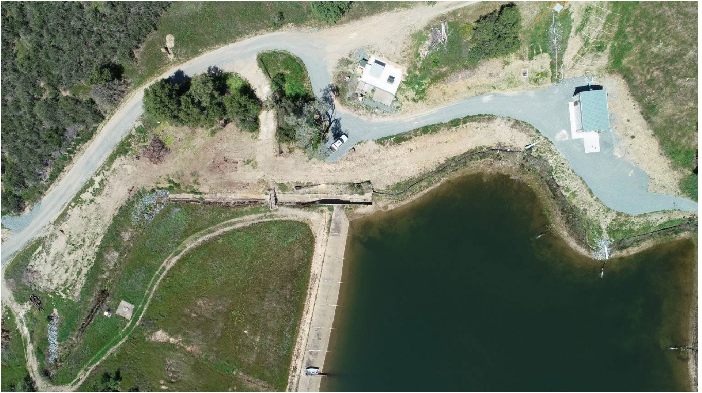
Electric equipment and transformer in top center, new hydroelectric powerhouse top upper right, lone reservoir in bottom right quarter with dam at bottom center
