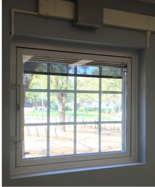
Figure 6: Electrical Wiring for the Internal Shade Motor
