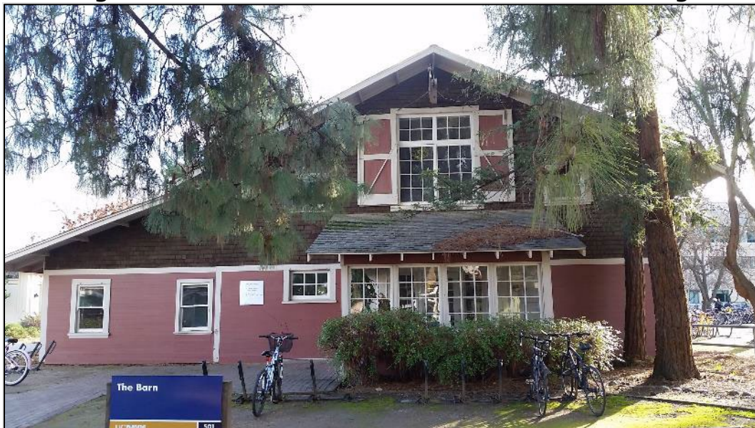
Figure 3: North Facade of the Demonstration Building
