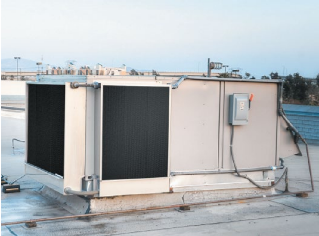
RTU with combined evaporative condenser air pre-cooling and ventilation air pre-cooling.
