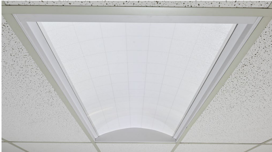
Figure 46: Volumetric LED Troffer Installed Into a Ceiling Grid in a Commercial Building
