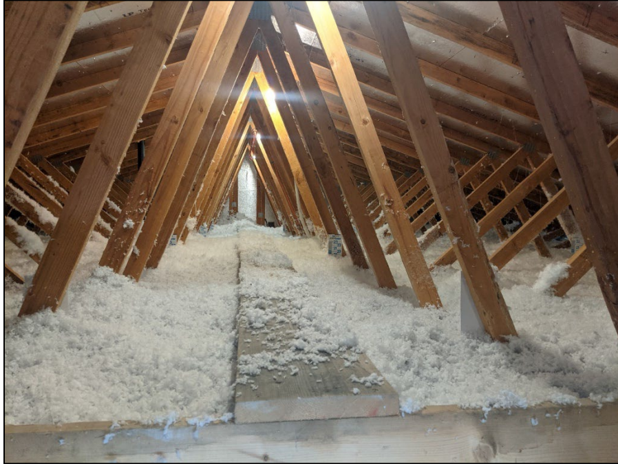
Figure 5: Attic Space Showing Deep Blown-In Insulation
