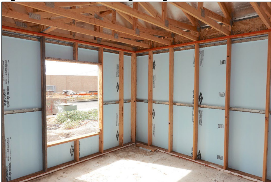
Figure 3: Advanced Framing During Construction Process.
