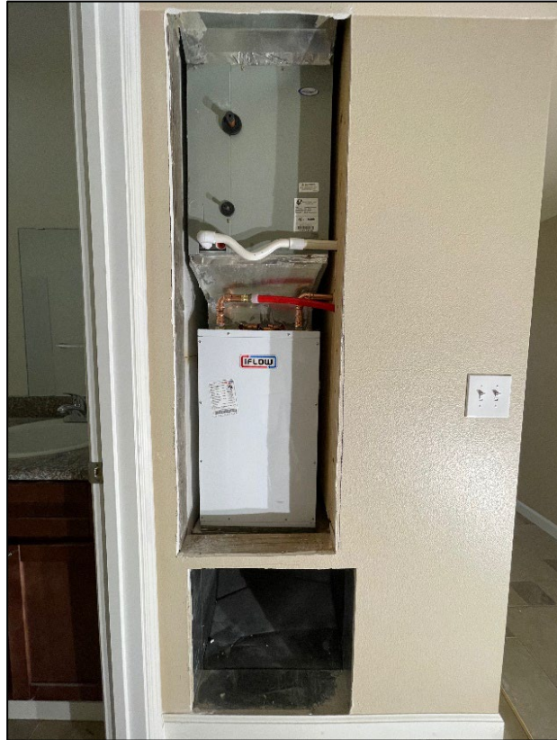
Figure 11: Combined Hydronic System in Mixed-Fuel Home
