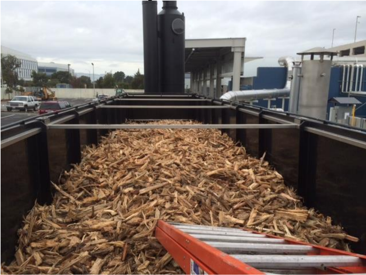
Biofilter with acid scrubber in background. Biofilter dimensions: length 42.64 feet, width 9.84, height 8.53, with media depth of 6.56 feet.
