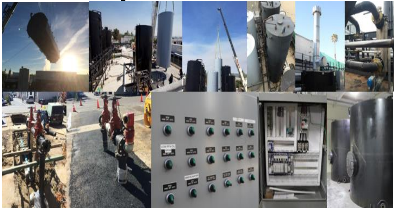
Figure 7: Phase Two of Construction
