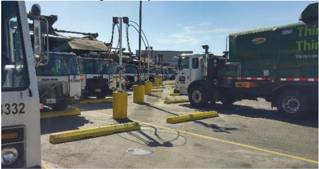
Figure 3. Completed Time Fill Line
