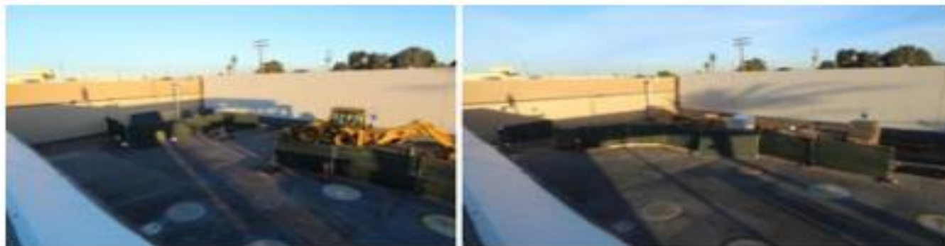
1 Feb - Beginning of excavation
