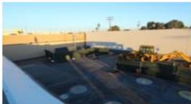
1 Feb - Beginning of excavation
