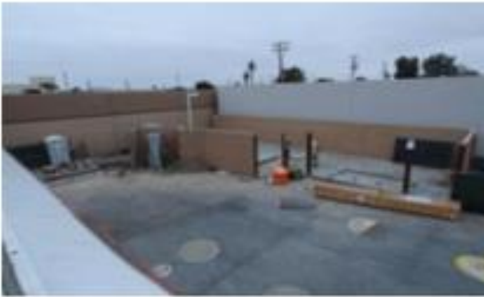
19 May - Prepared for equipment delivery
