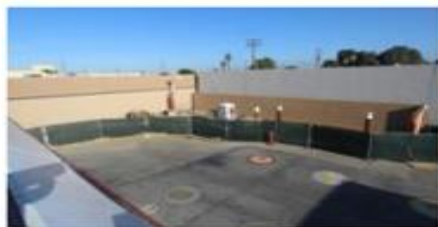
29 Mar - Walls and posts complete
