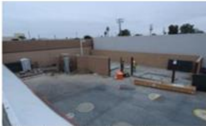
19 May - Prepared for equipment delivery
