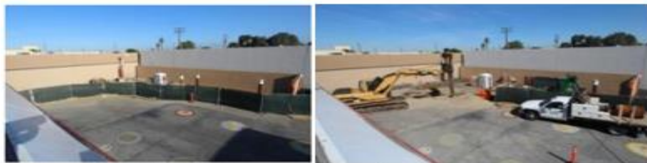
29 Mar - Walls and posts complete
