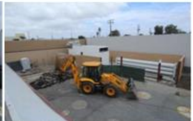
20 May - Excavation of fueling area
