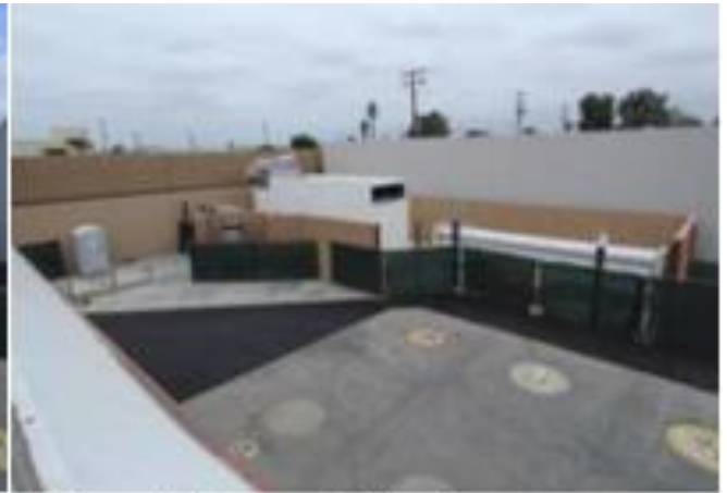
30 May - fueling area finished
