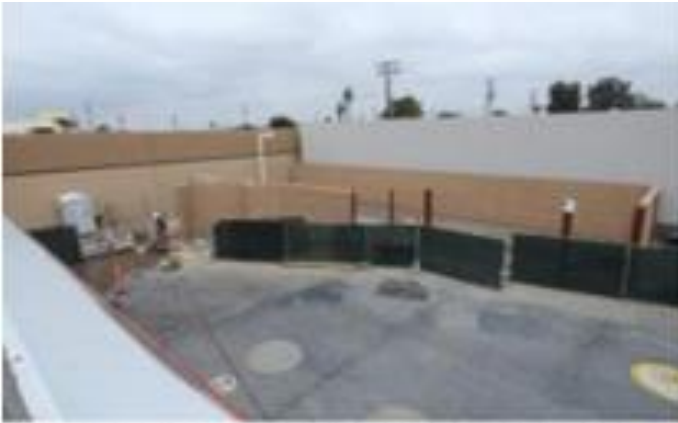
17 May - Prepared for equipment foundations
