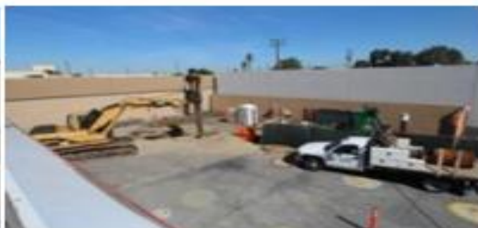
20 Apr - Canopy foundation excavation
