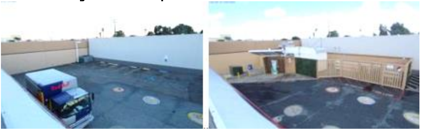
Figure 3: Site comparison: Pre- & Post- HRS installation
