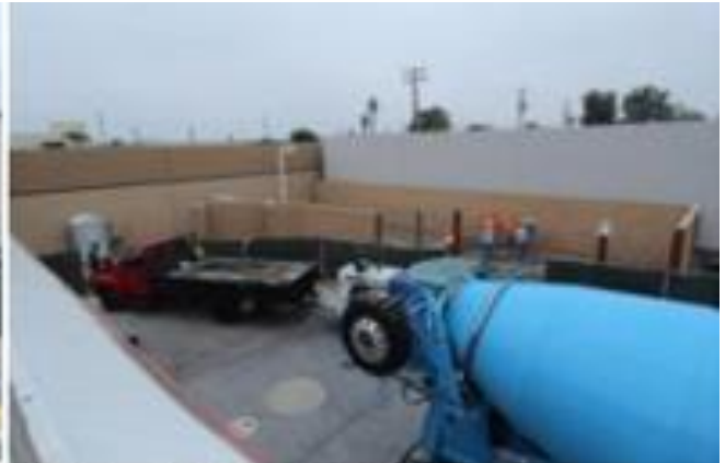
18 May - Equipment foundations
