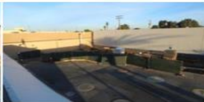
23 Feb - Beginning construction of back wall
