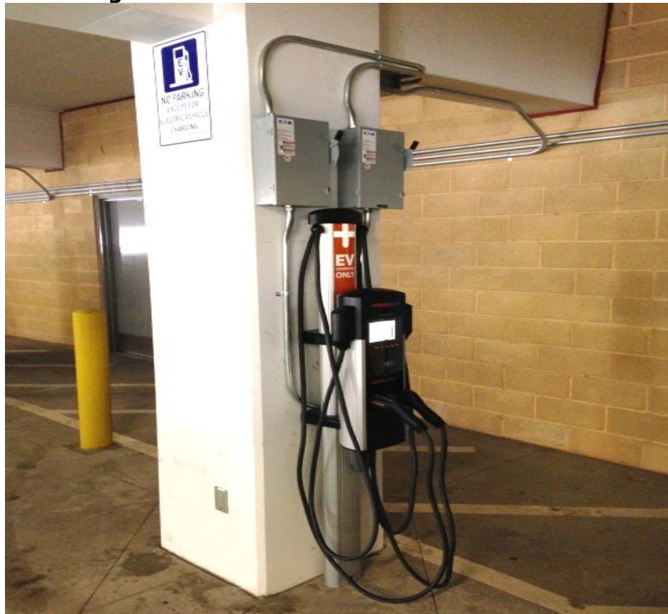
Figure 11: Electrical Disconnect Installation
