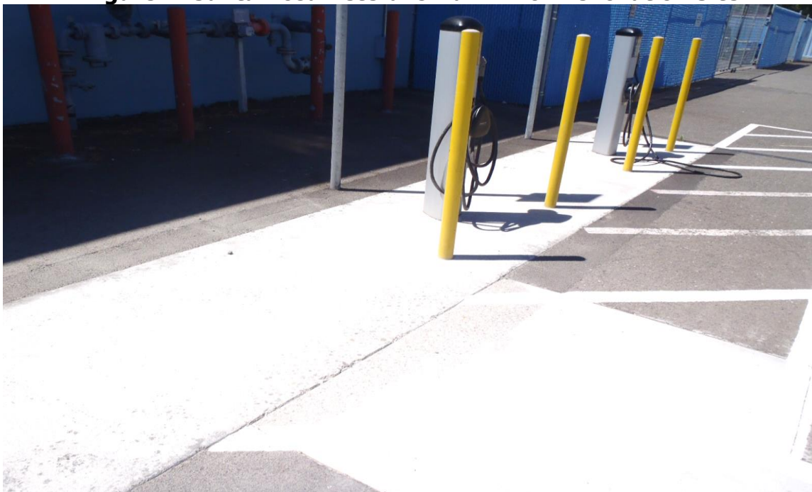
Figure 2: Santa Rosa Veterans Hall Minor Renovation Site
