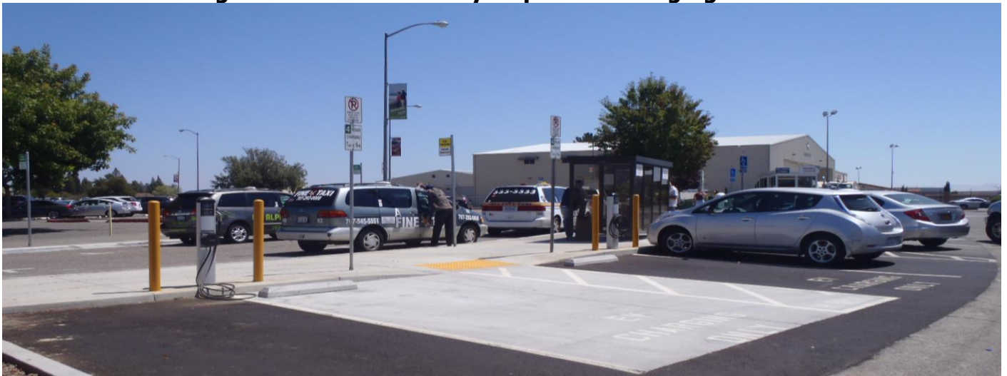
Figure 5: Sonoma County Airport EV Charging Site
