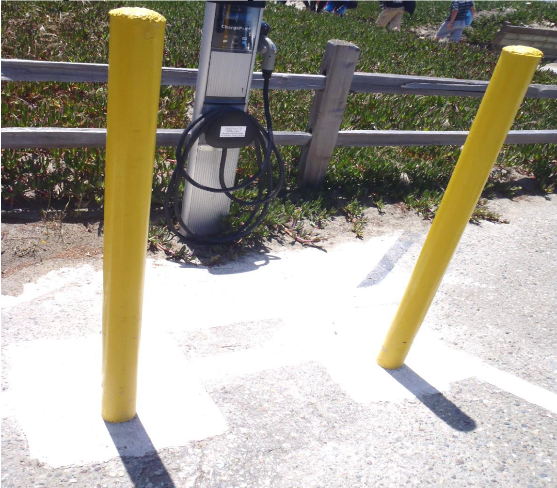
Figure 3: Doran Beach Regional Park Minor Renovation Site
