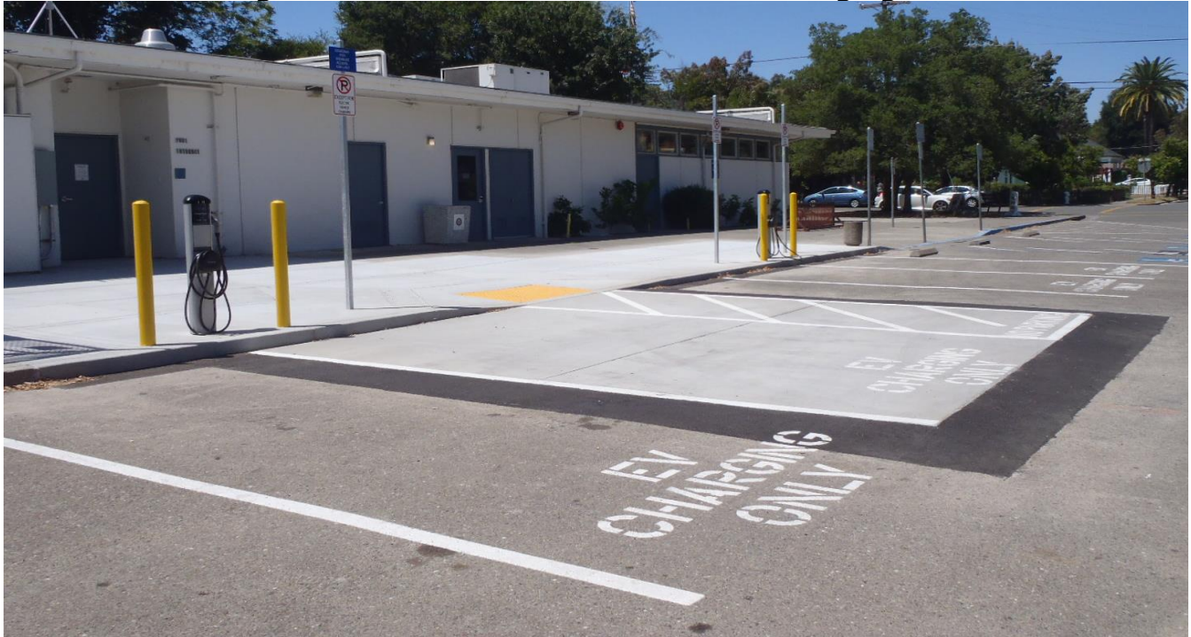
Figure 6: Cloverdale Veterans Hall EV Charging Site
