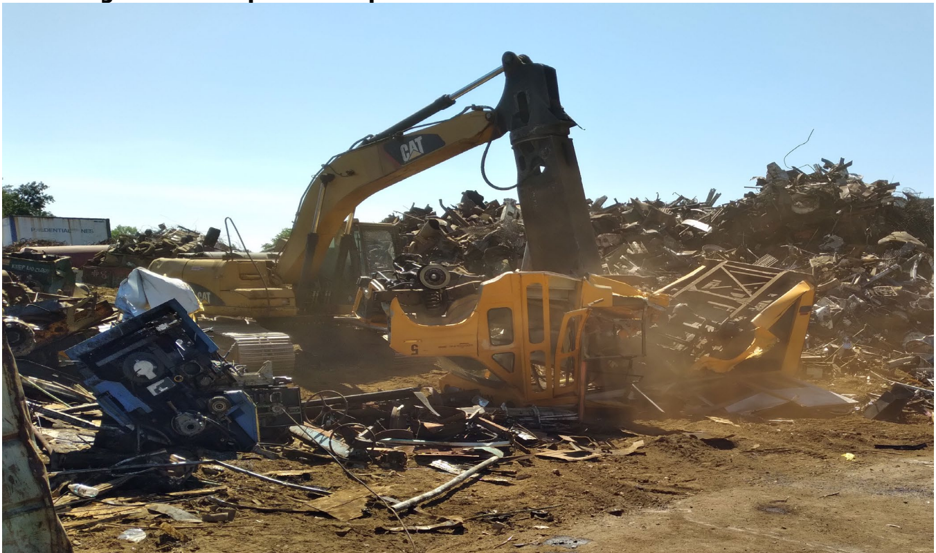
Figure 2: Example of Acceptable Method to Dismantle Vehicle Chassis
