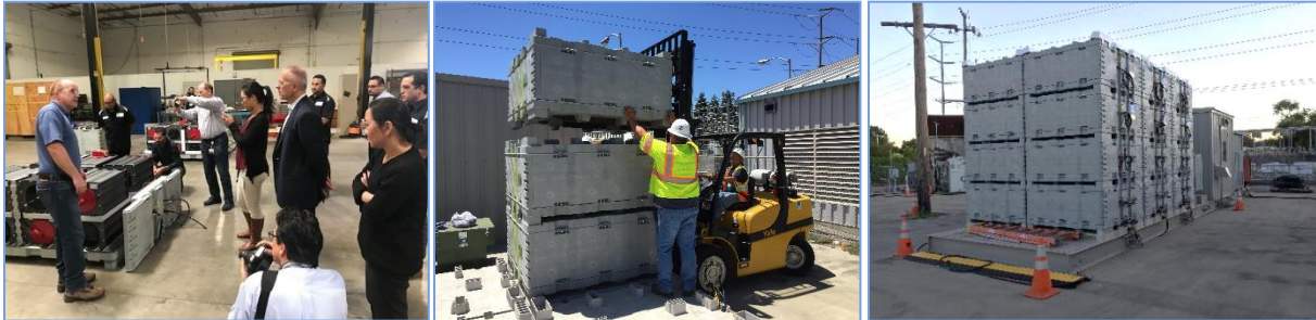
Figure 19: Integration, Installation, and Commissioning of the 75kW AC-integrated System for Testing With SDG&E at the San Ramon Technology Center
