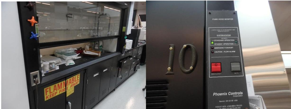
Photo on the left: Fume Hoods and Existing Fume Hood Phoenix Controls.
