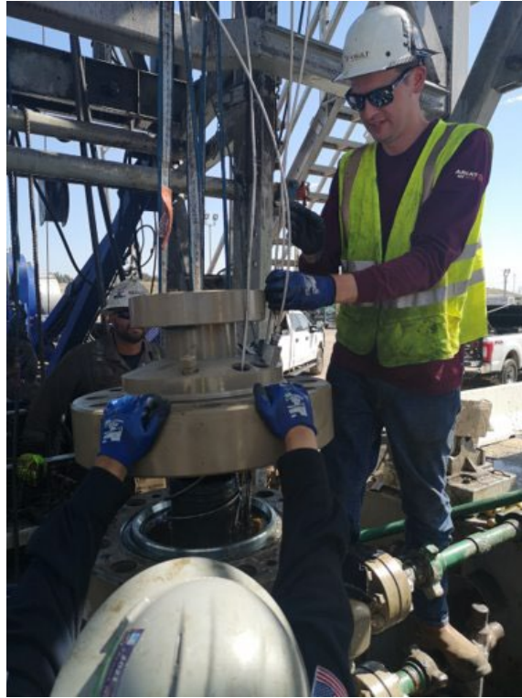
Figure 6: Fiber Optics Installation at PG&E’s McDonald Island Gas Storage Field
