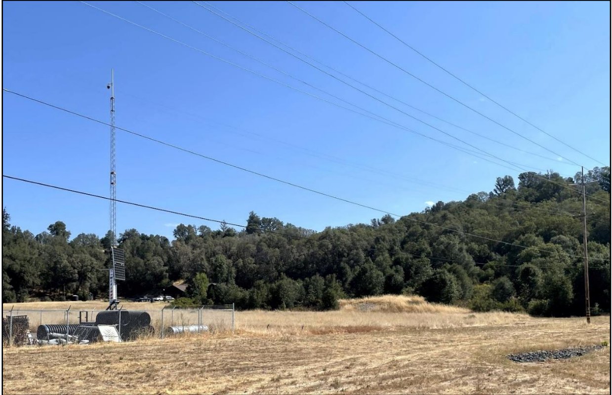
Figure 5.1-1. Existing View of Power Block 1 Site
