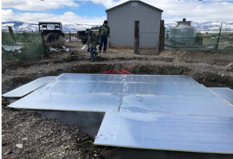
Figure 50: Insulation of hot spring.
