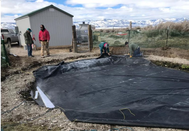
Figure 51: Rubber tarp for second layer of insulation.
