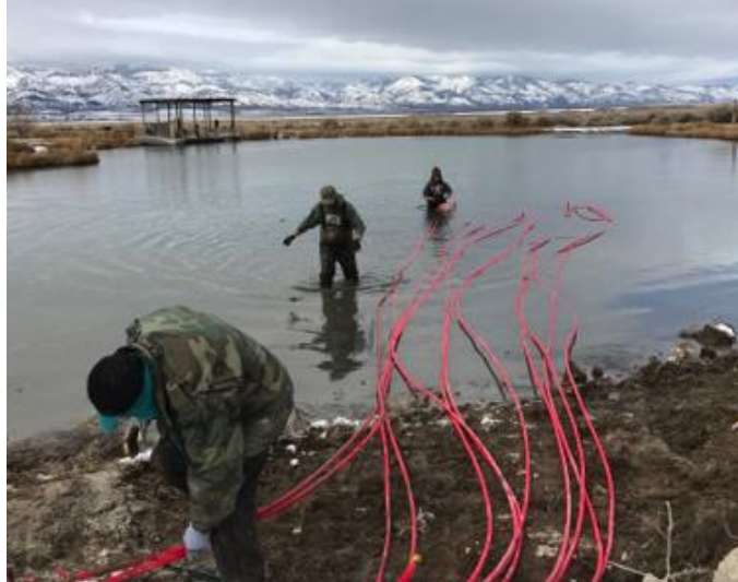
Figure 46: Installation of cold water loops.
