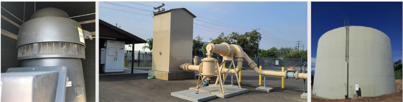
**A variable-speed pump, shelters for pump/controls, and a storage tank at Tubeway Station 32**
