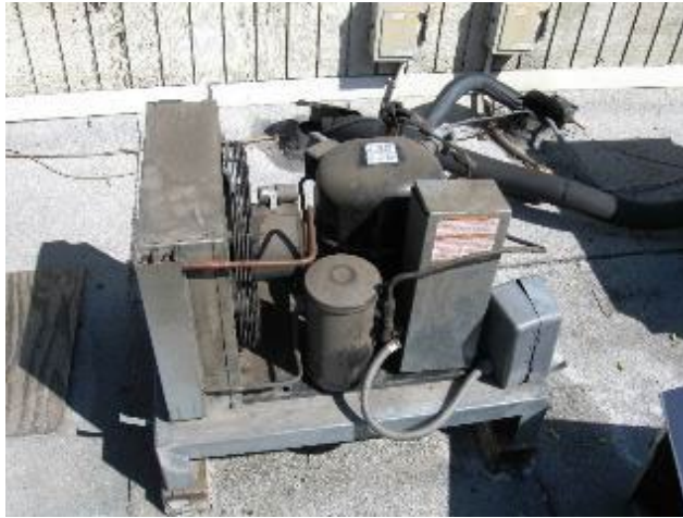
Figure 116. Remote Refrigeration Rack with Single Compressor.
