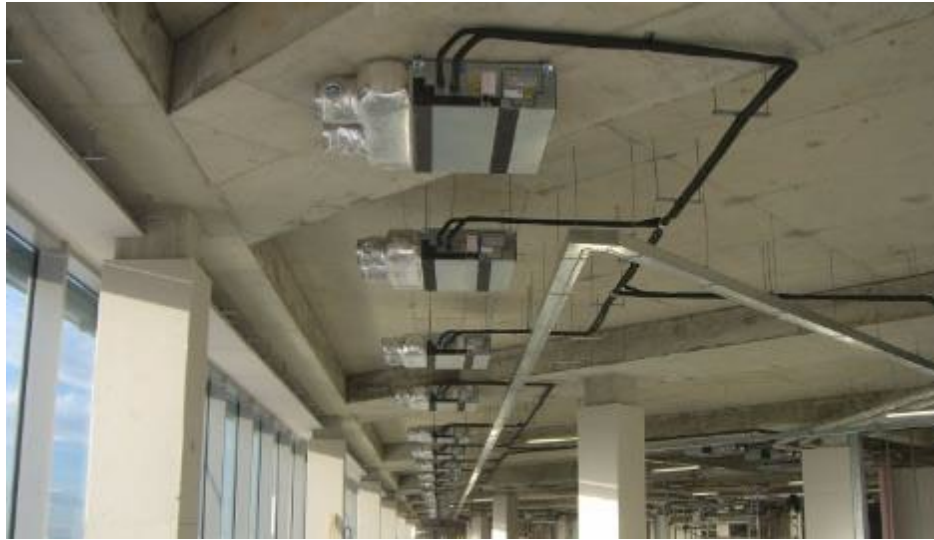
Figure 81. Split System Indoor Fan Coil without Ducting.
