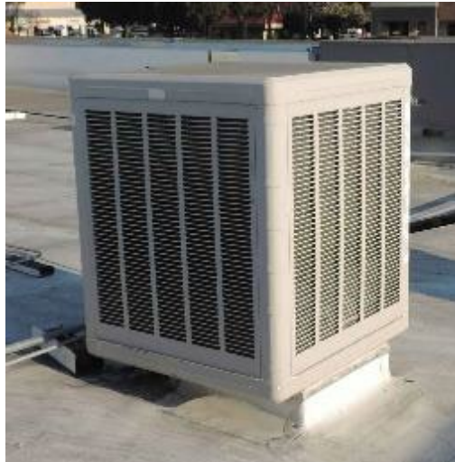
Figure 88. Roof Mounted Evaporative Cooler.
