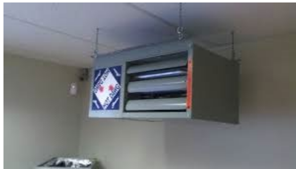
Figure 62. Electric Heater for Room.
