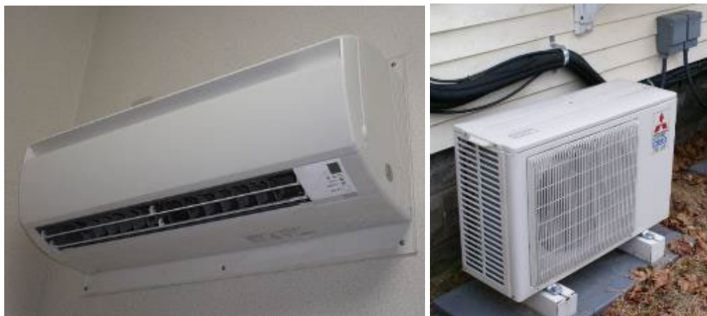
Figure 60. Indoor Fan (left) and Outdoor part (right) of Ductless Mini-Split Heat Pump.
