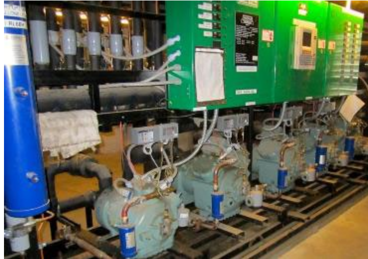
Figure 114. Central or Remote Refrigeration Rack with Multiple Compressors.
