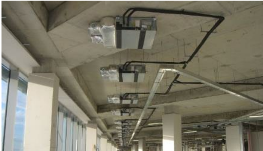
Figure 58. Split System Indoor Fan Coil without Ducting.
