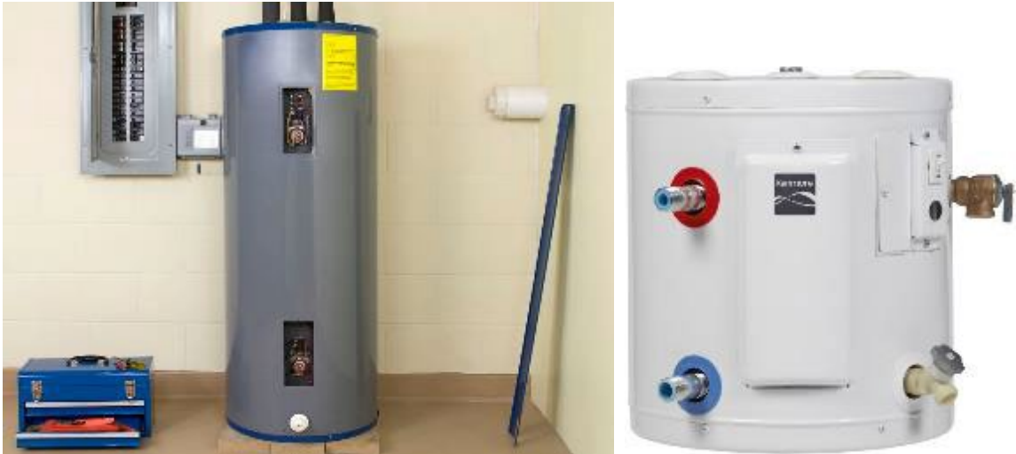
Figure 93. Electric Water Heaters.
