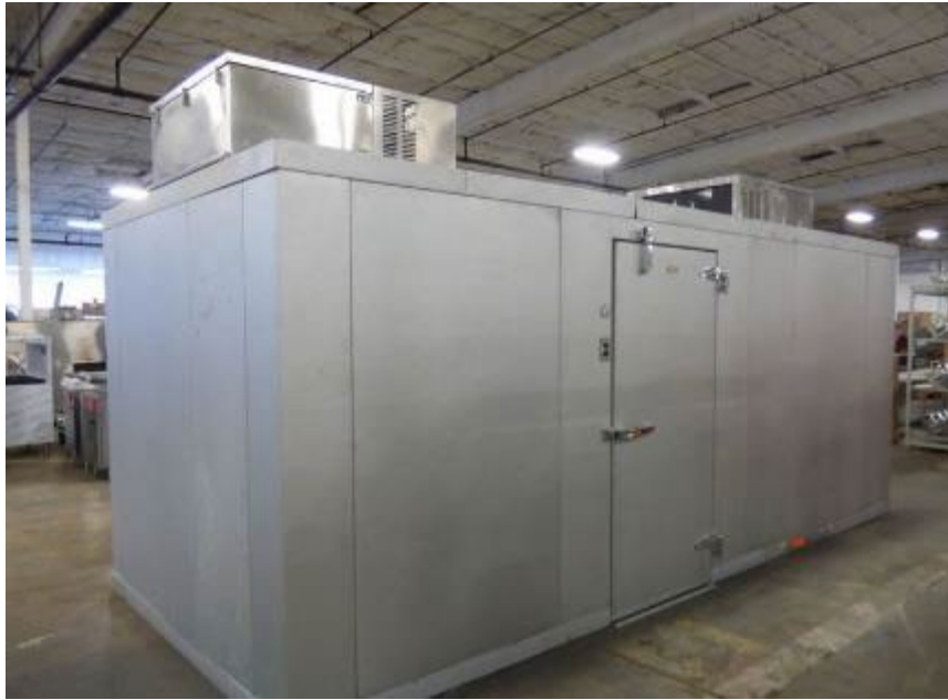
Figure 125. Self-contained Walk-In Cooler or Freezer, Compressor on roof of the cooler.
