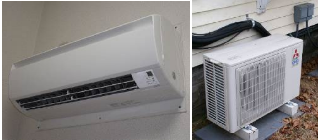
Figure 84. Indoor Fan (left) and Outdoor part (right) of Ductless Mini-Split Heat Pump.
