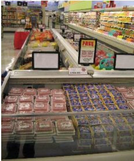
Figure 119. Refrigerated Coffin Cases served by Central/Remote Compressor Rack (not in picture).
