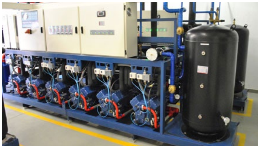
Figure 115. Central or Remote Refrigeration Rack with Multiple Compressors.
