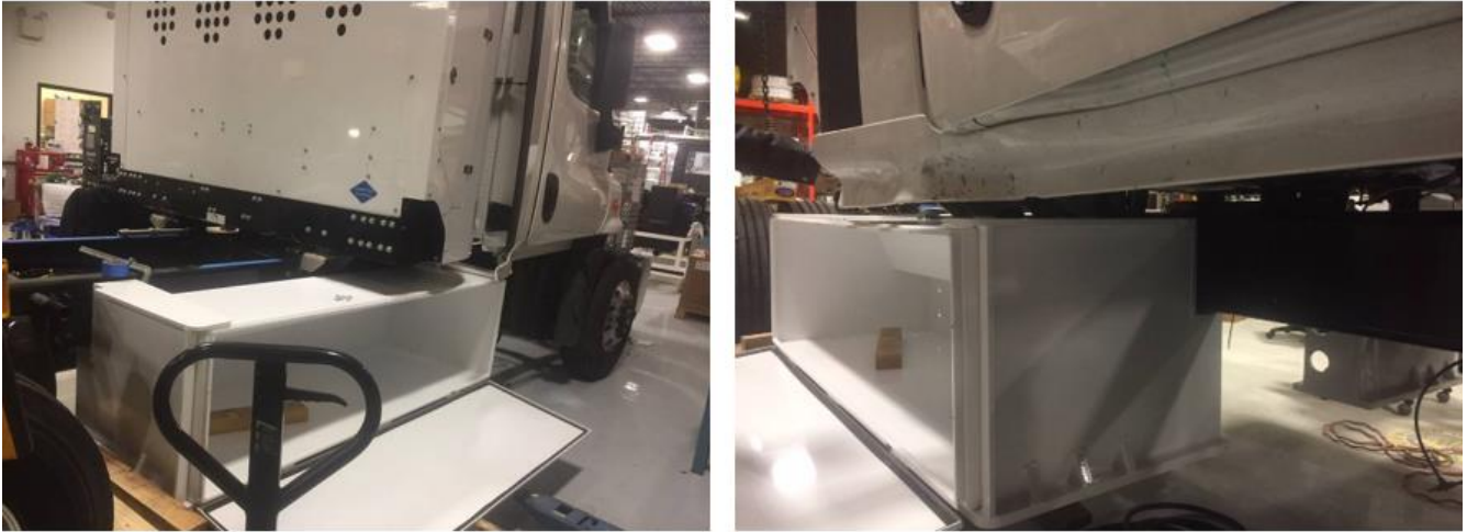
Figure 32: High Voltage Battery Bracket Installation
