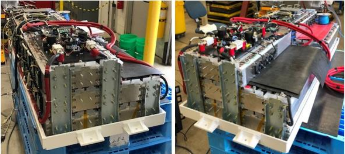
Figure 35: High Voltage Battery Packs Installation
