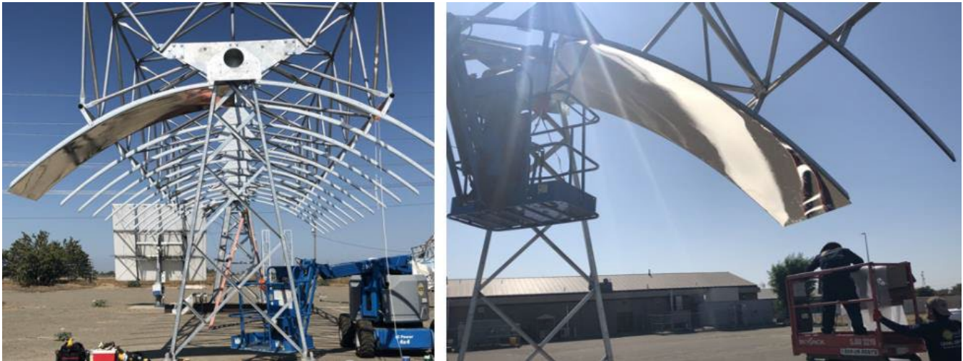
Figure 23: Installation of first half mirror panel on the parabolic ribs
