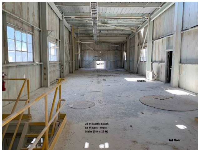
Figure 10: Space on the third level of building housing the kettle
