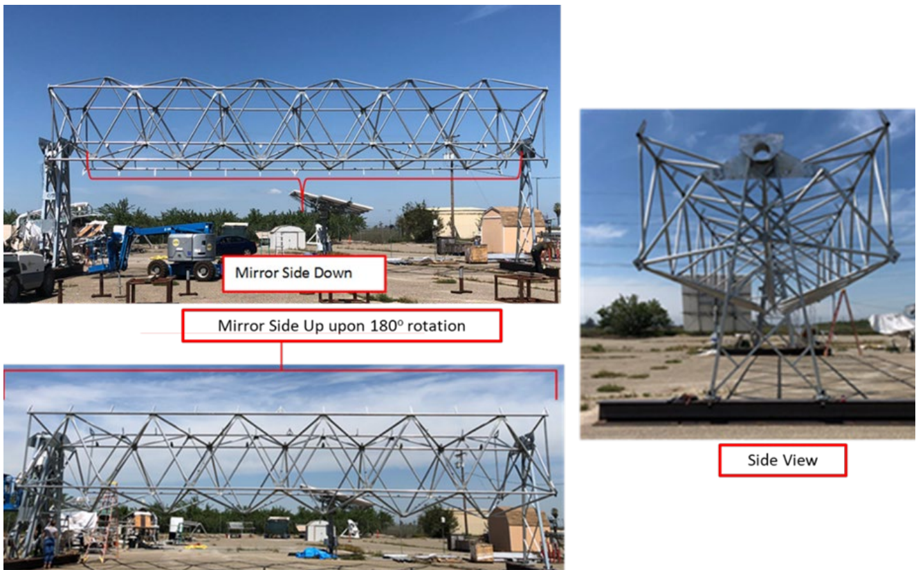
Figure 22: The mirror support space frame assembled and rotated at UCM
