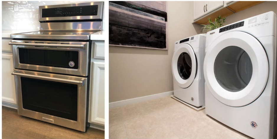
Figure 1: Induction Cooktop (Left) and Heat Pump Dryer (Right) Installed in All-Electric, Zero Net Energy Community in Irvine, California
