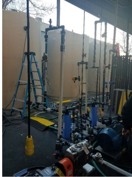
Figure 23: Installation and Plumbing of Storage Tanks for Process Fluids
