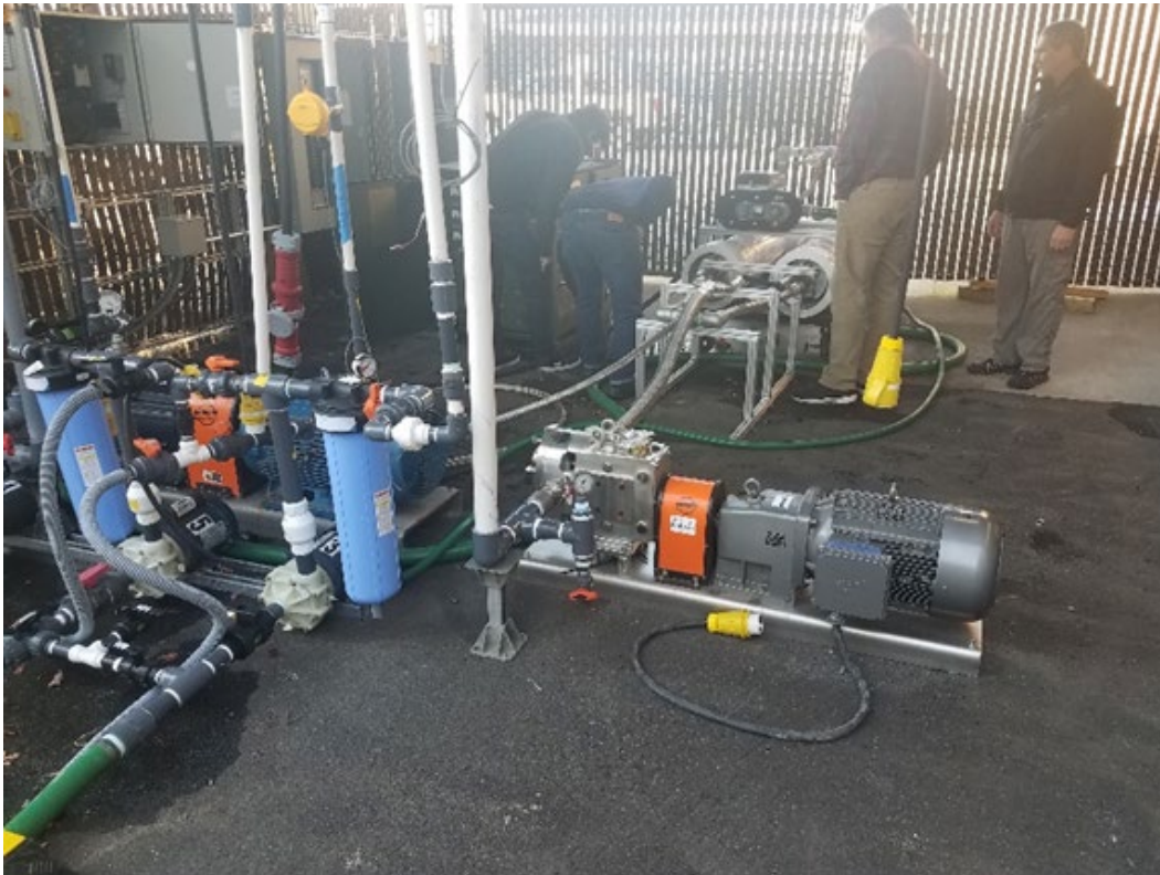
Integration of two membrane modules completed.
