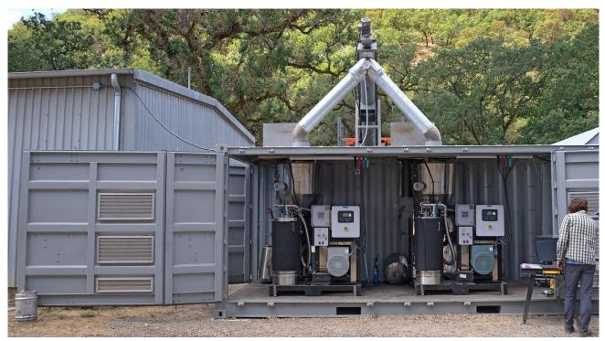
Figure 5: 50 kW PP30 Microgrid Container In-Field Installation
