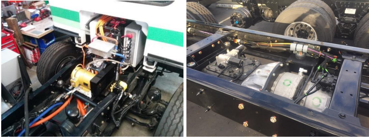
Figure 17: PCAS and MDS Mounted into the Chassis
