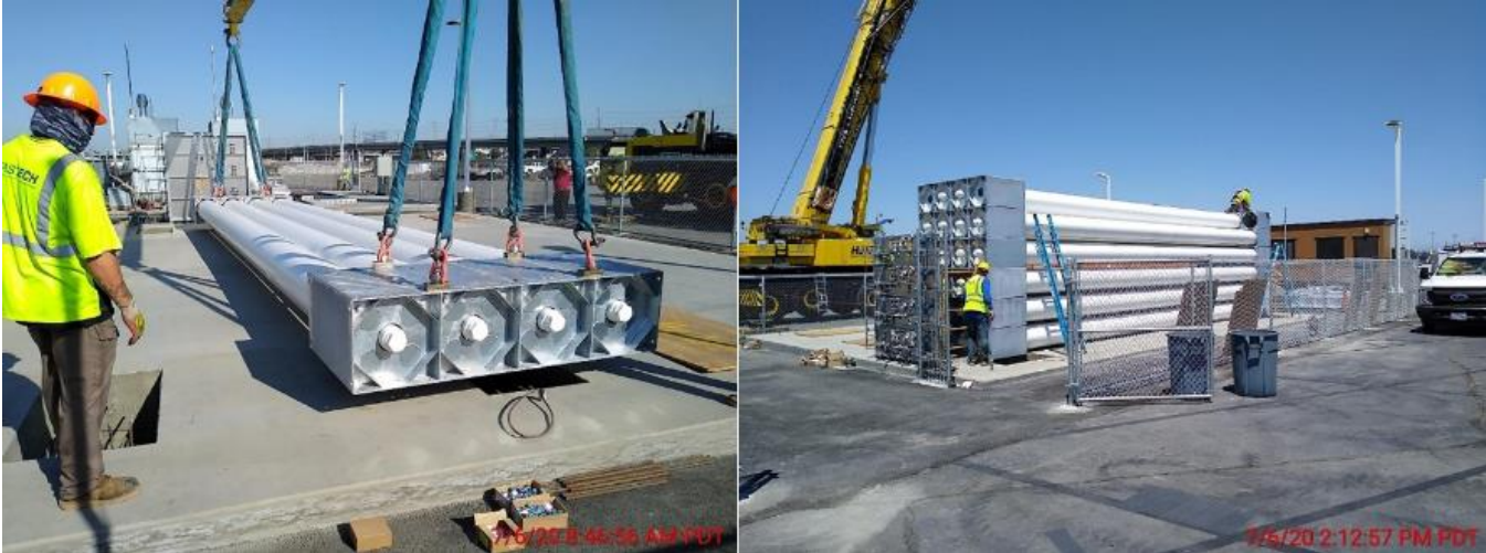
Figure 3. Field Assembly of Storage Module
