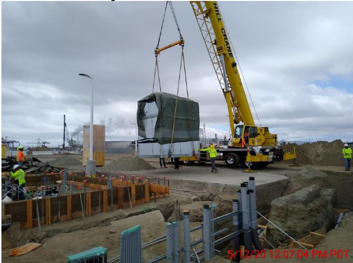
Figure 4. Lift and Set of Station Module
