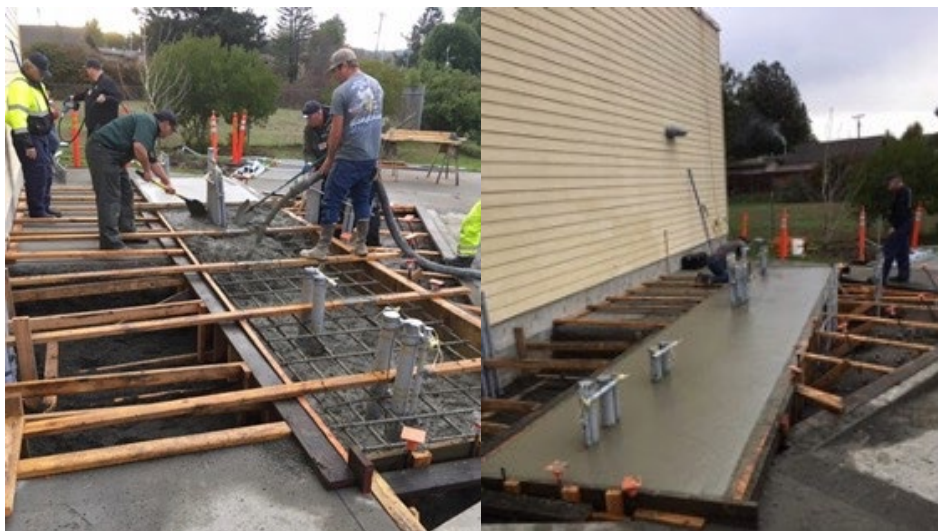
Staff pouring concrete for the main equipment slab.
