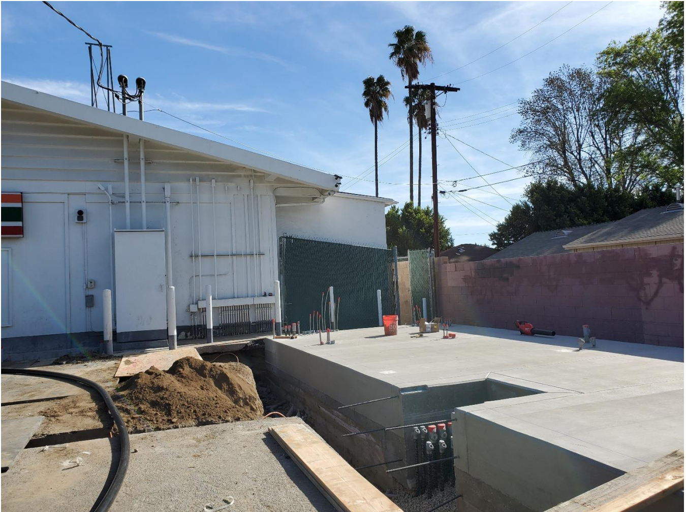
Figure 6: Completed Equipment Pad at the Mission Hills Station
