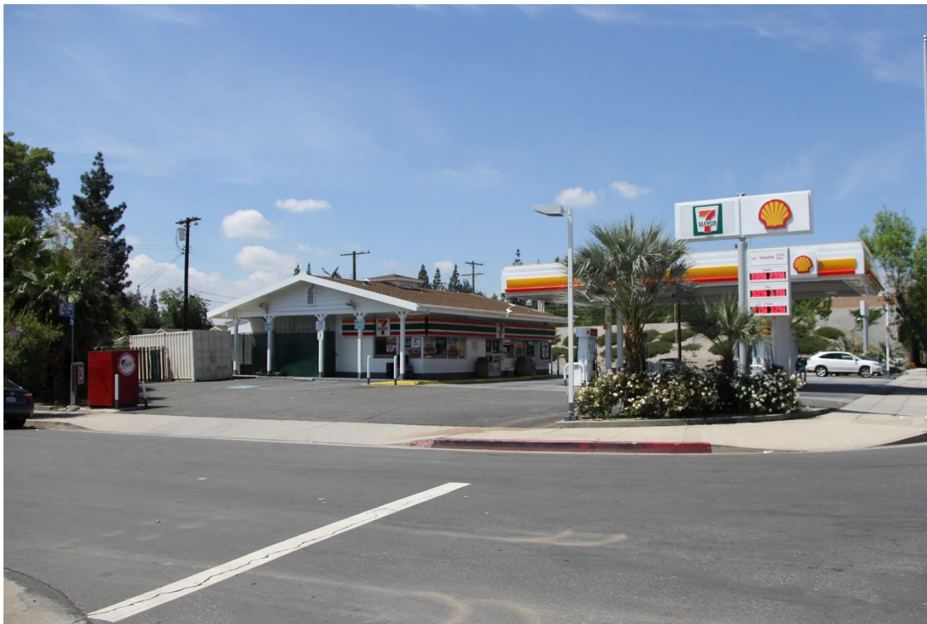
Figure 2: Property View During Acquisition Phase
