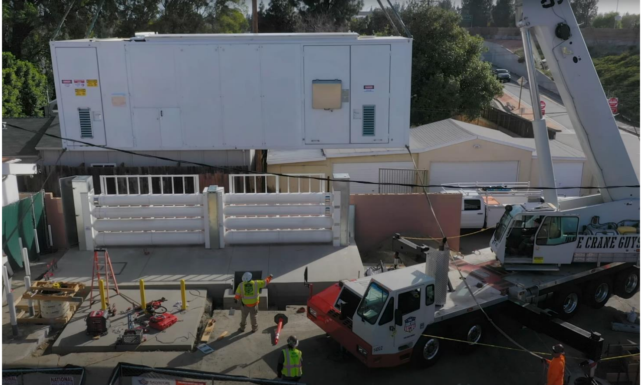
Figure 7: Linde Equipment Installation at the Mission Hills Station
