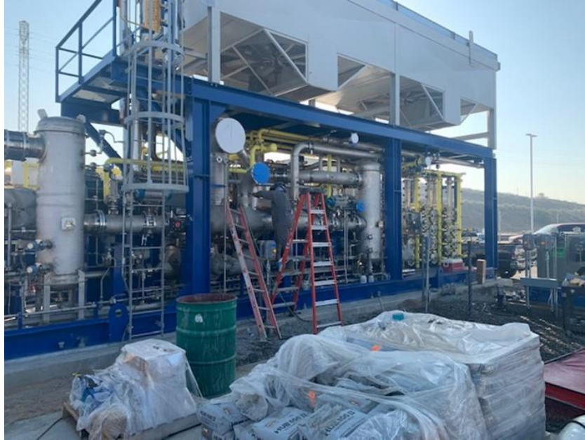
Figure 14: Piping Installation at Biomethane Upgrader
