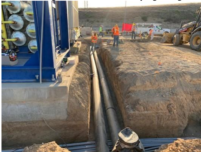
Figure 15: Underground Biomethane Piping Being Installed
