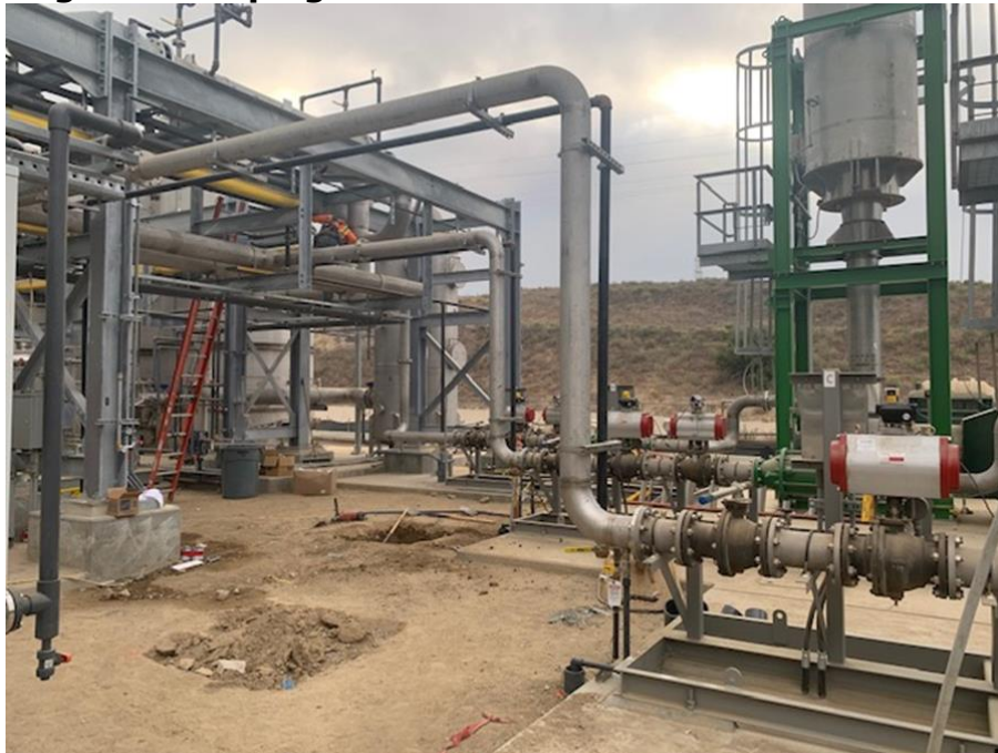
Figure 16: Piping Connections to Gas Train Assemblies
