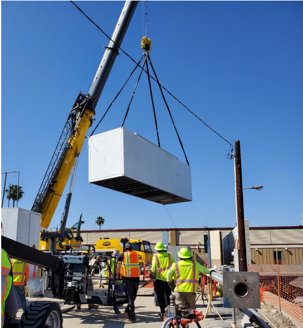
Figure 8: Crane lifting hydrogen ground storage unit off delivery truck.
