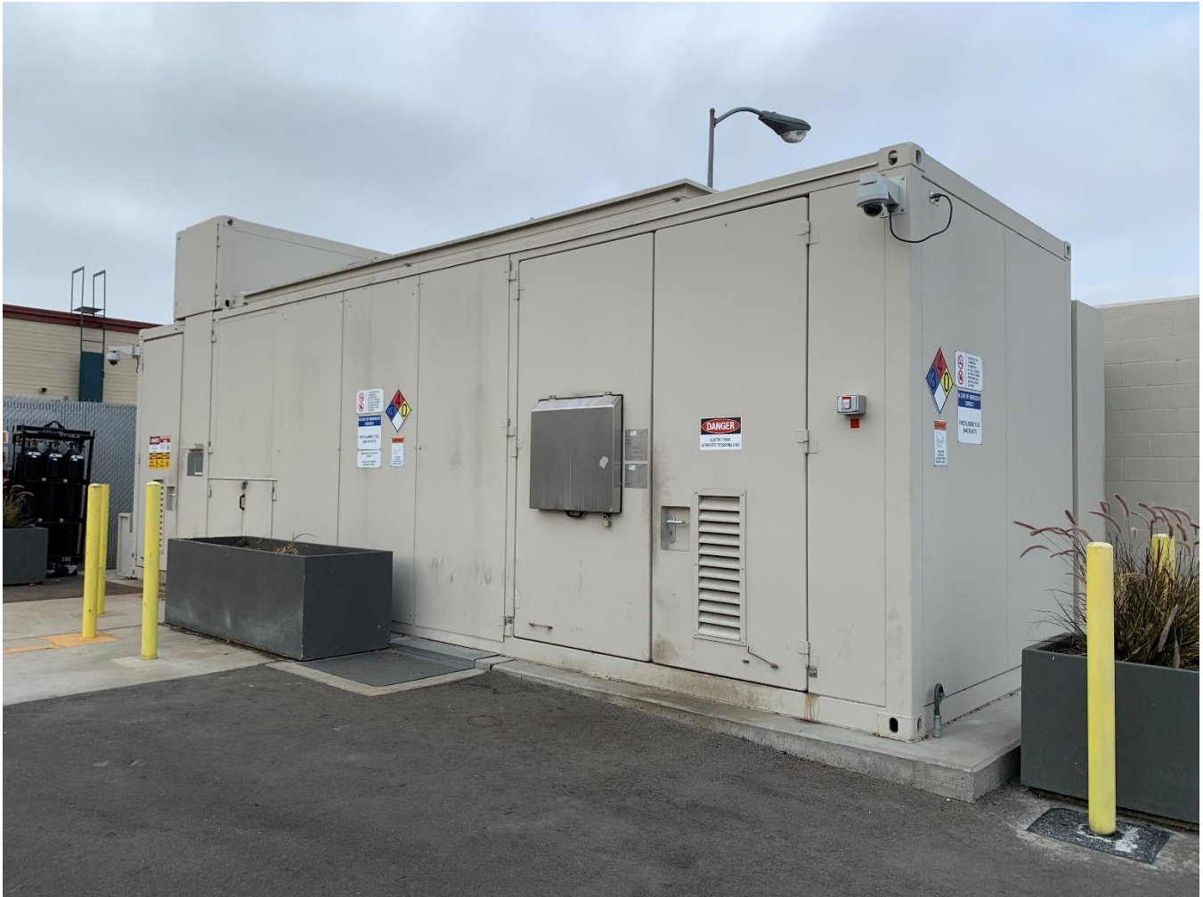
Figure 4: Installed Linde Unit (Compressing and Dispensing Equipment).
