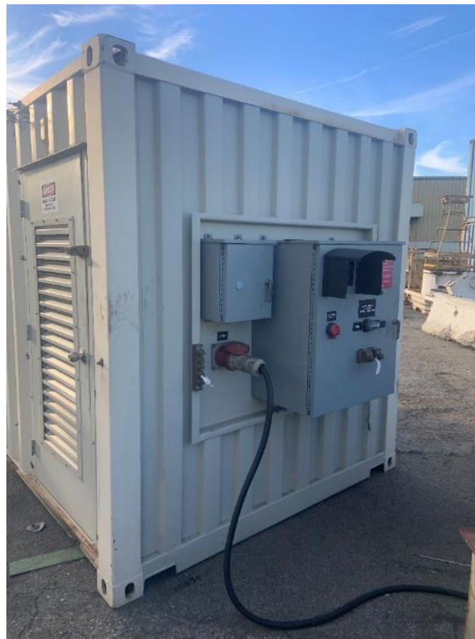
Figure 21 - Battery Pack Connector Panel
