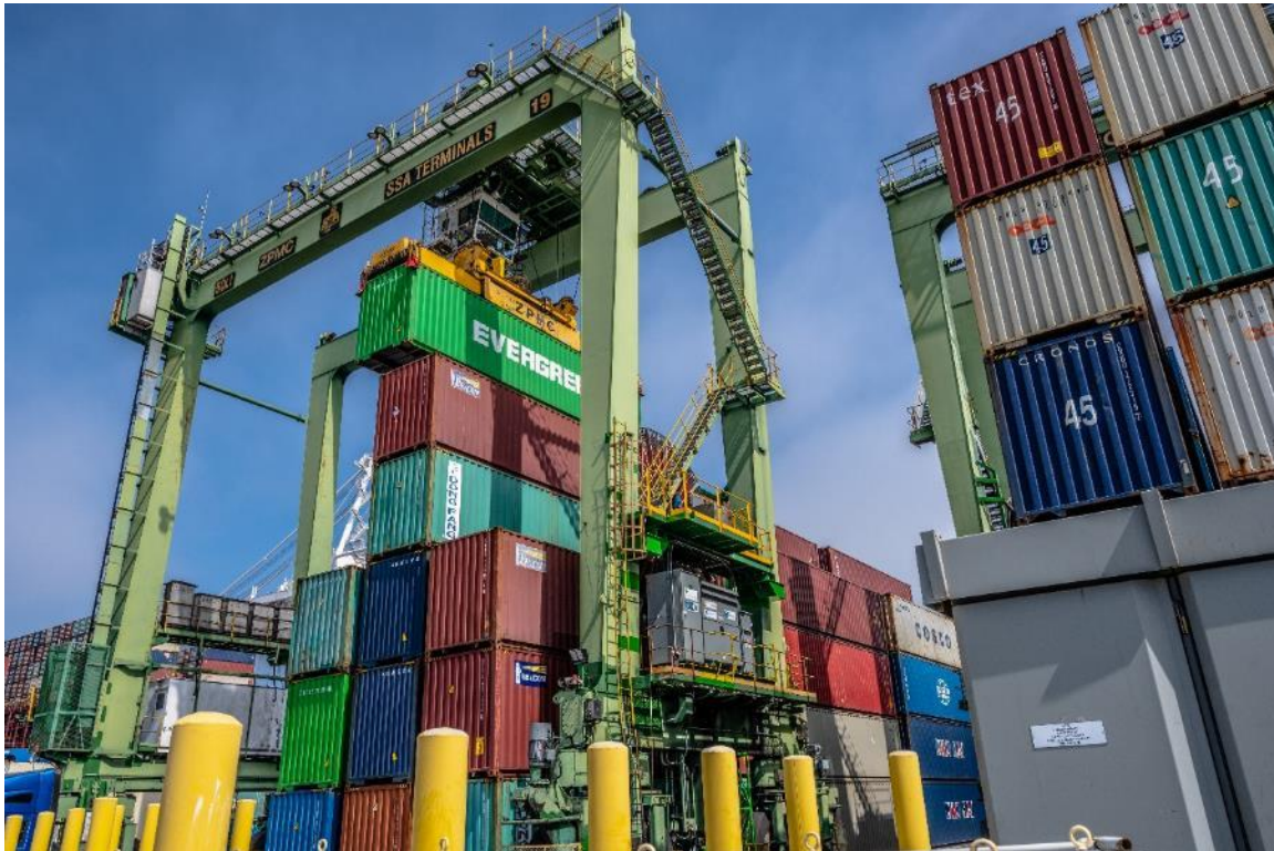
Figure 19 - eRTG 9, SSA Crane 19 (Final Conversion)
