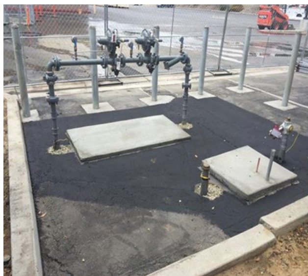
Figure 12: Site Gas Service Upgrades
