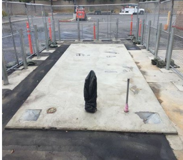
Figure 13: Concrete Pad for the Product
