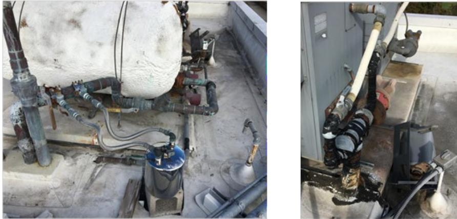
Figure C-4: Existing Storage Tank Water Piping and Boiler Gas Piping
