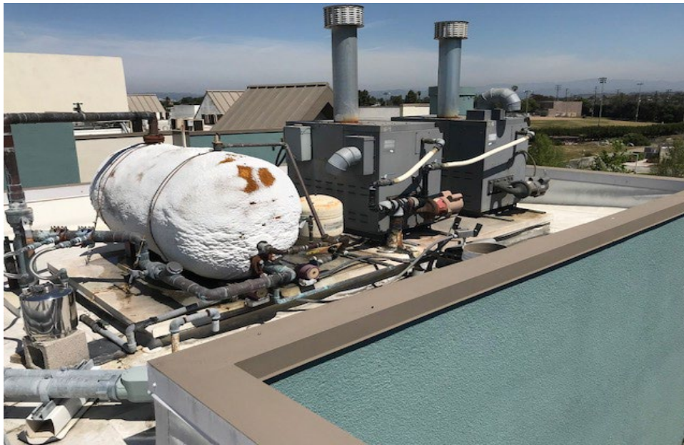
Figure 2: Boilers and Storage Tank on the Roof
