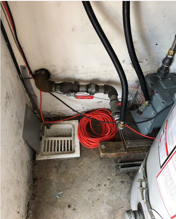
Figure E-4: Water Heater Gas Meters Installed at Site #1 (Left) and Site #2 (Right)
