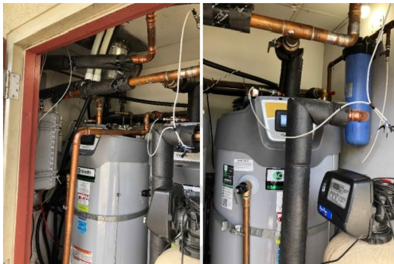
Figure 18: Replacement Water Heaters at Site #1
