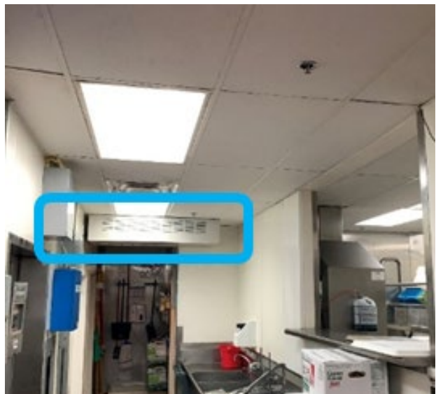
Figure 30: Location of Fan Coil Unit at Site #1 (Left) and #2 (Right, Highlighted)
