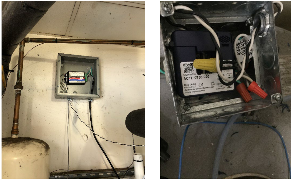
Figure E-5: Water Heater Power Meters Installed at Site #1 (Left) and Site #2 (Right)
