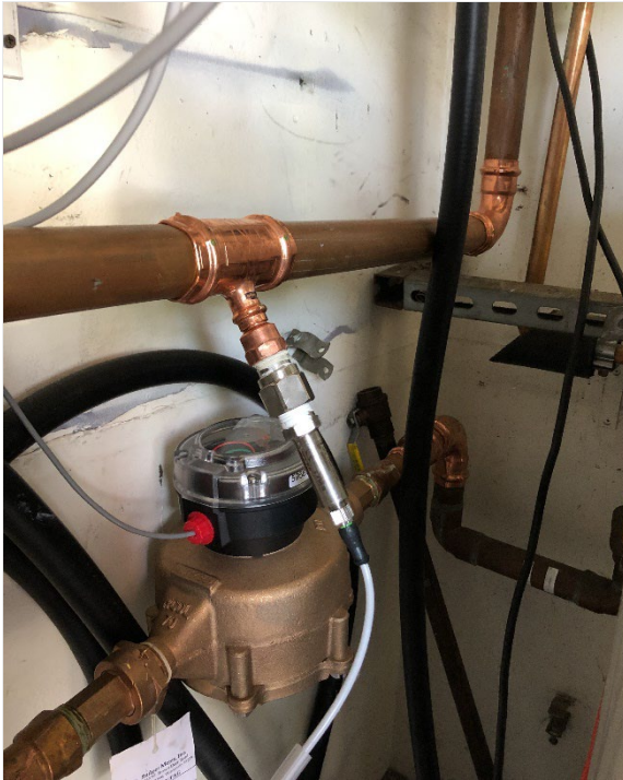
Figure E-3: Water Meter Installed at Site #1 (Left) and Site #2 (Right)
