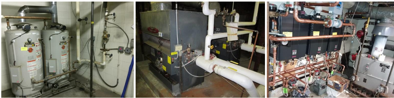
Figure 1 Typical Commercial Water Heating Installations from Prior Field Studies, Storage-type, Boiler & Indirect Storage Tank, and Tankless-Type Equipment (Left to Right)
