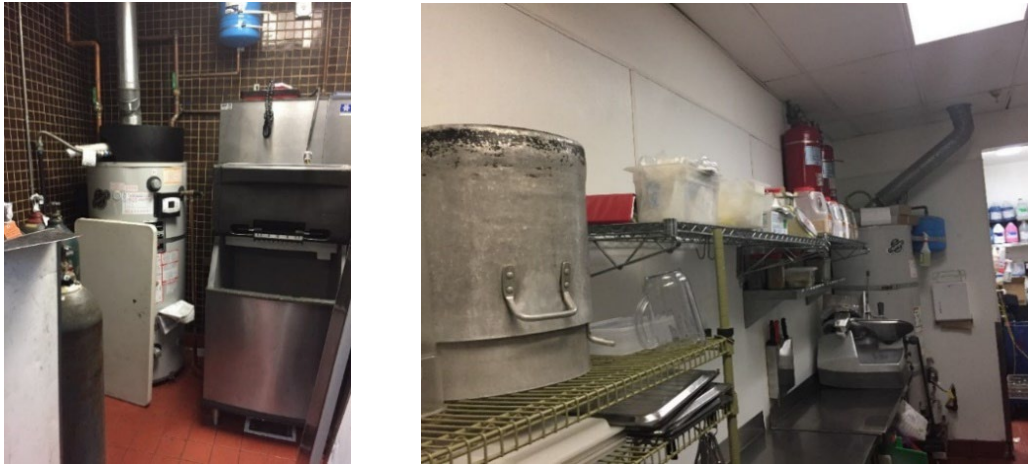
Figure A-10: GWHs at Inspected Sites Without Space for Adjacent Indirect Storage Tank
