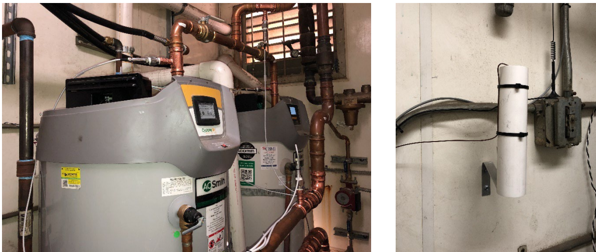
Figure E-2: Hot/Cold Water and Mechanical Room Air Temperature Measurements at Site #2
