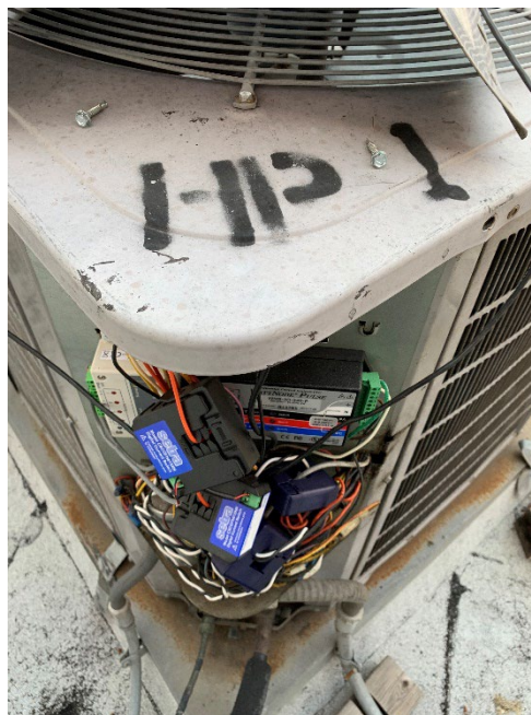
Figure D-3: WattNode and Switches Installed on a Heat Pump (Cover Removed)
