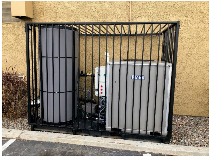
Figure 27: Photos of Initial GHP Skid Placements Including Anti-Vandalism Cages at Site #1 (Left) and Site #2 (Right)
