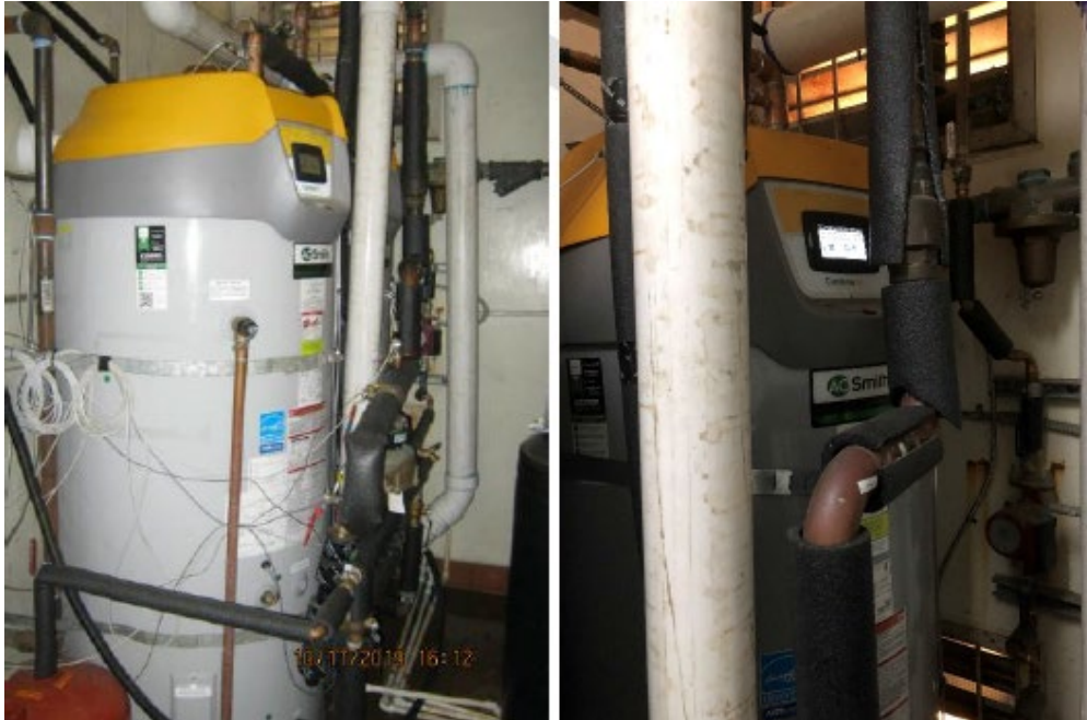
Figure 19: Replacement Water Heaters at Site #2
