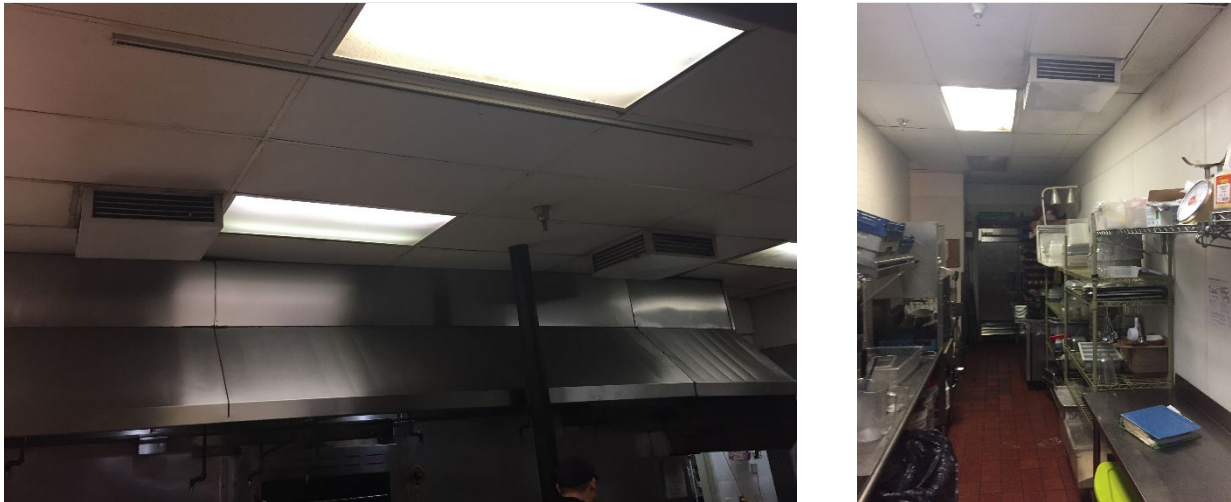
Figure C-13: Distribution in Kitchen Area above Cook Line (Left) and Back Kitchen Area (Right)
