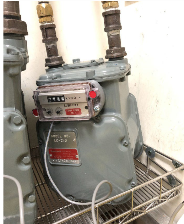
Figure E-4: Water Heater Gas Meters Installed at Site #1 (Left) and Site #2 (Right)
