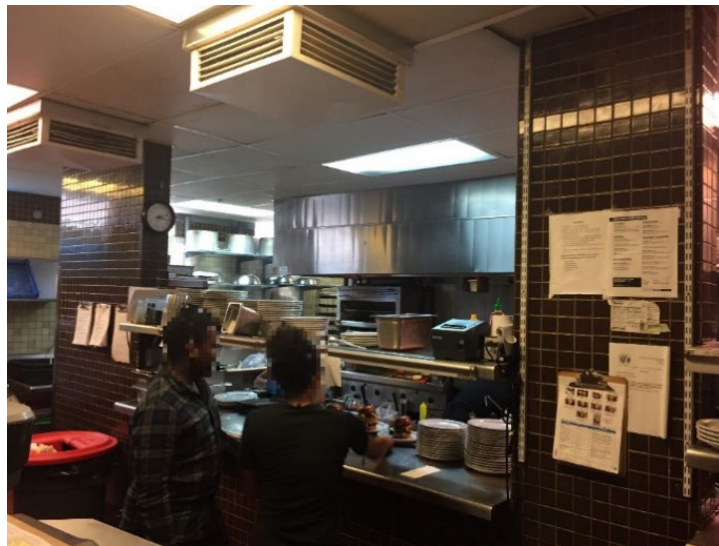
Figure C-6: Location of Two Supply Air Diffusers in Kitchen
