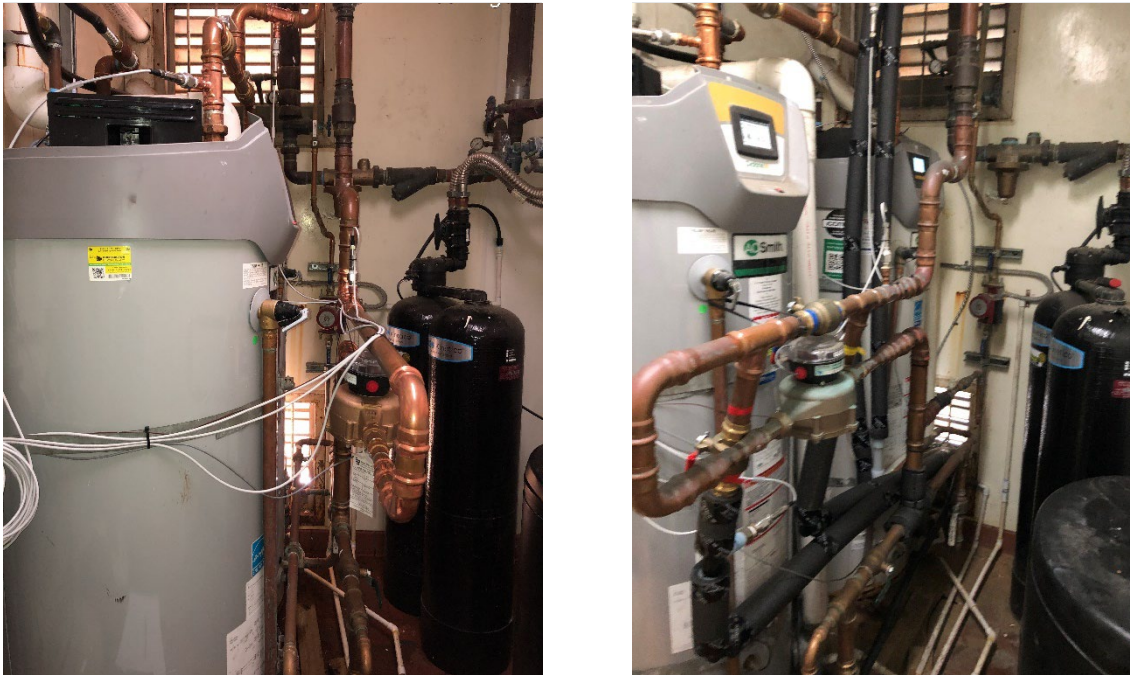
Figure 31: Before and After Integrated Gas Heat Pump System Commissioning at Site #2
