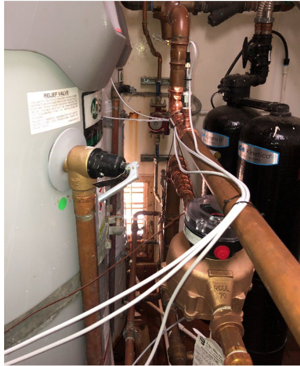
Figure E-3: Water Meter Installed at Site #1 (Left) and Site #2 (Right)
