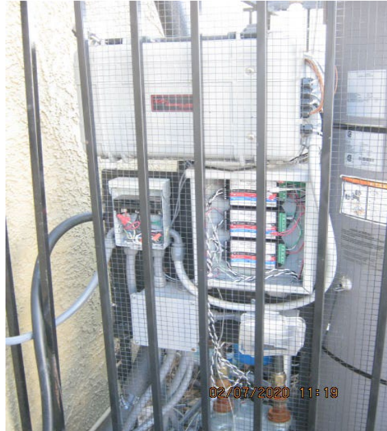
Figure D-11: Opened Enclosures from Tampering
