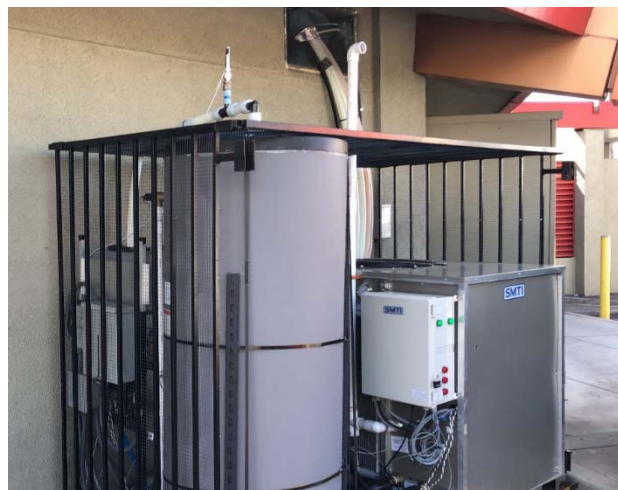
Figure 1: Commercial Gas Heat Pump Skid Package Installed at Host Site
