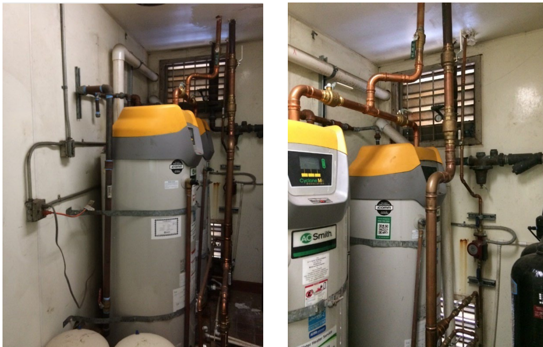
Figure C-41: Indoor Water Heaters at Site #2A
