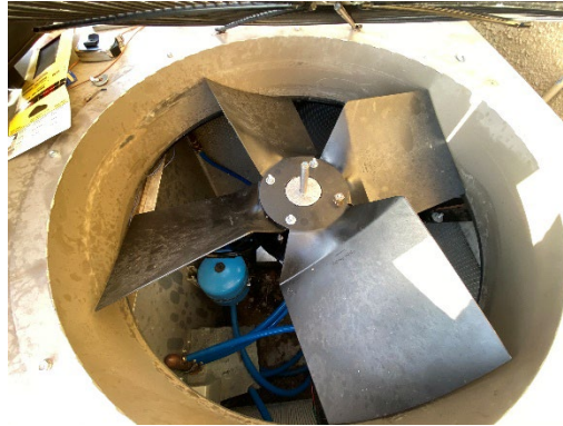
Figure D-7: Evaporator Fan Replacement
