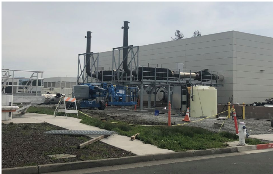
SRC units on CHP units (1.1 MW each) to reduce emissions
