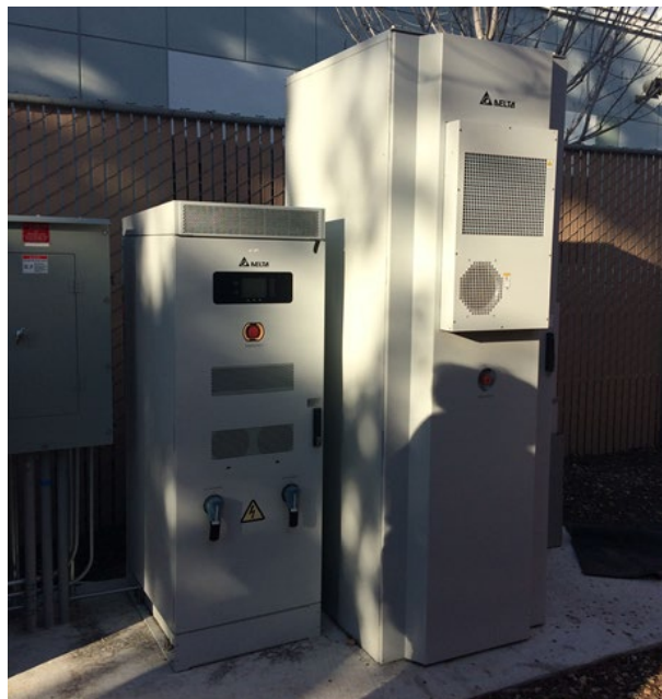
Delta's battery system (right) and power conditioning system (left) in the fire station yard
