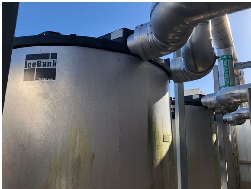
One of a dozen legacy 3,200-ton/hour ice storage tanks
