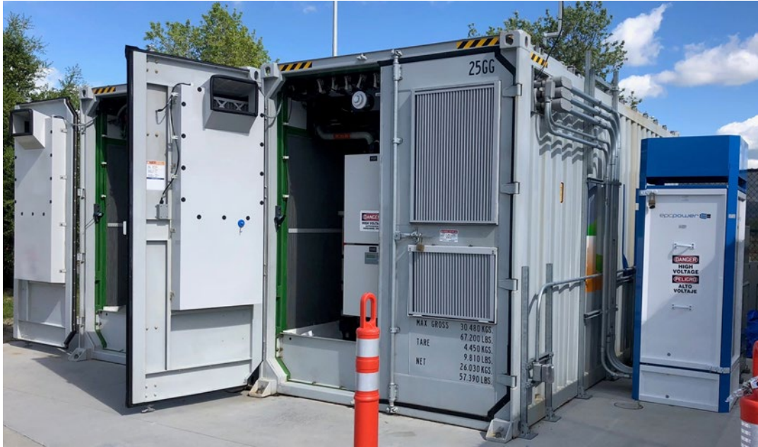
Figure 21: Vanadium Flow Battery Storage System and Inverter
