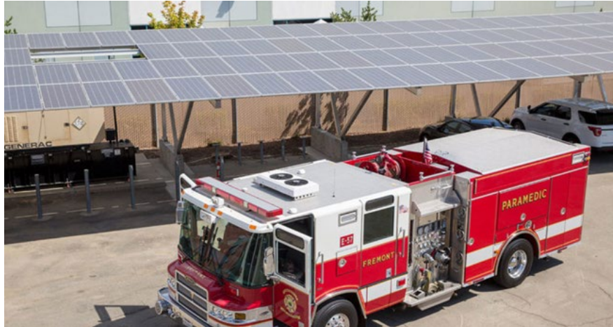
43-kW carport solar array at one of the Fremont Fire Stations.
