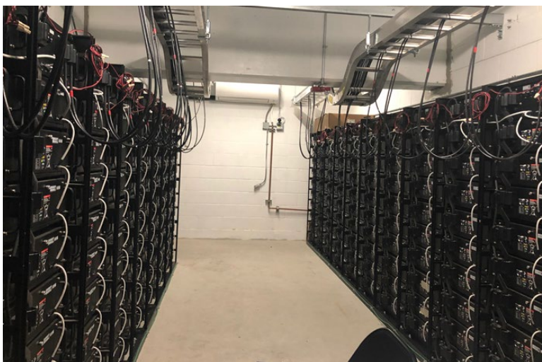
Shipping container-sized 250-kW/1-MWh battery energy storage system
