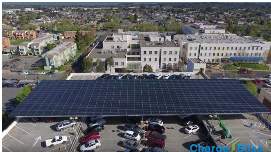
Aerial photo of the parking garage adjacent to Kaiser Permanente, including the 250-kW top-level solar array
