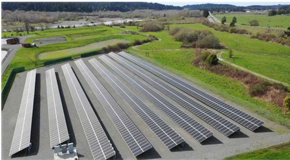
420-kW AC PV ground-mounted array at Blue Lake Rancheria
