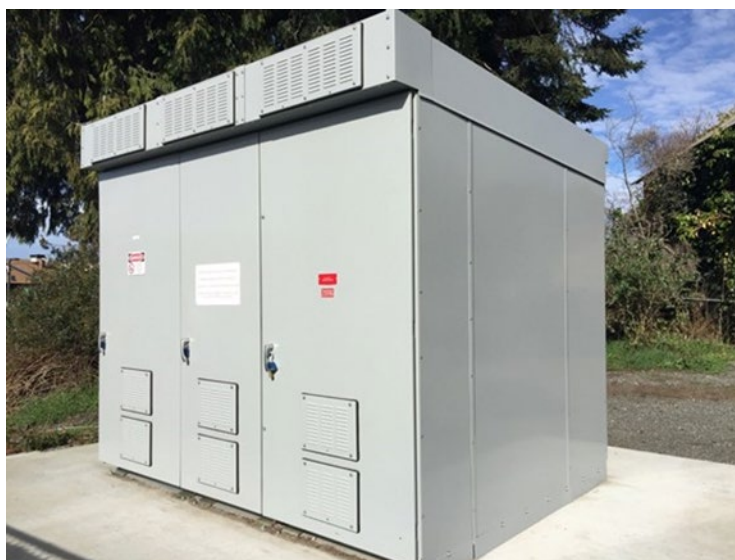
Point of common coupling (PCC) switchgear enclosure housing the PCC breaker, PCC battery system, and communications system
