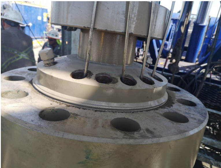
Top left: Optical fiber cable is hung by a sheave to help installation. Top right: Optical fiber cables are bonded by hose clamps at the bottom of the well above the packer. Bottom left: Optical fiber cables passed through the well head. Bottom right: Optical fiber cables and splicing were secured at the junction near the wellhead.
