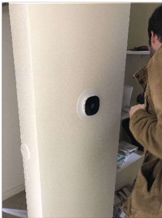
Figure 31: Installation of Smart Thermostats for Demand-Charge Management in Firebaugh, California
