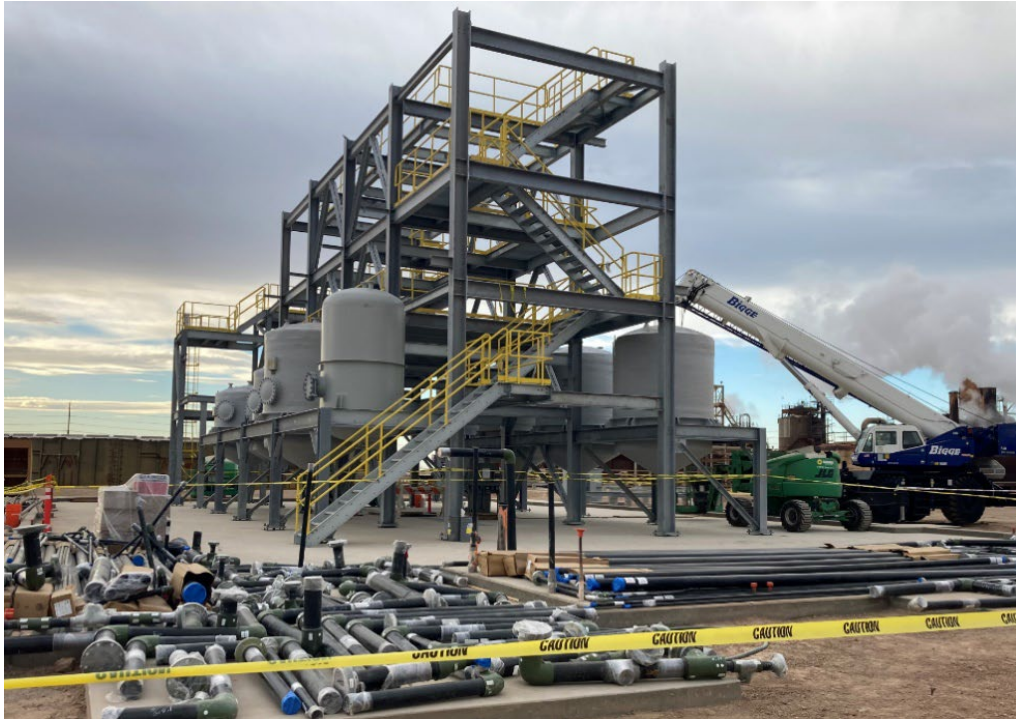
Figure 6: Nine Vessels Installed at the LRD Facility
