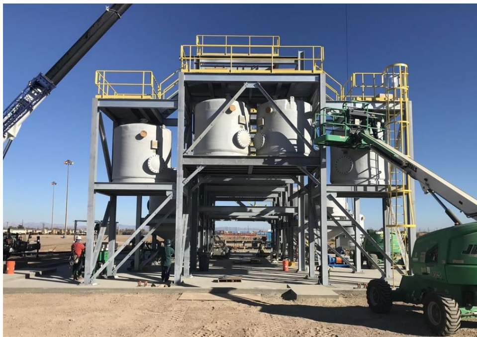
Figure 5: Four Reactor Tanks Set at the LRD Facility
