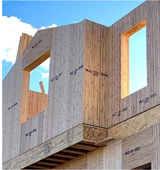
A PCTV building being erected using BamCore prefabricated structural panels
