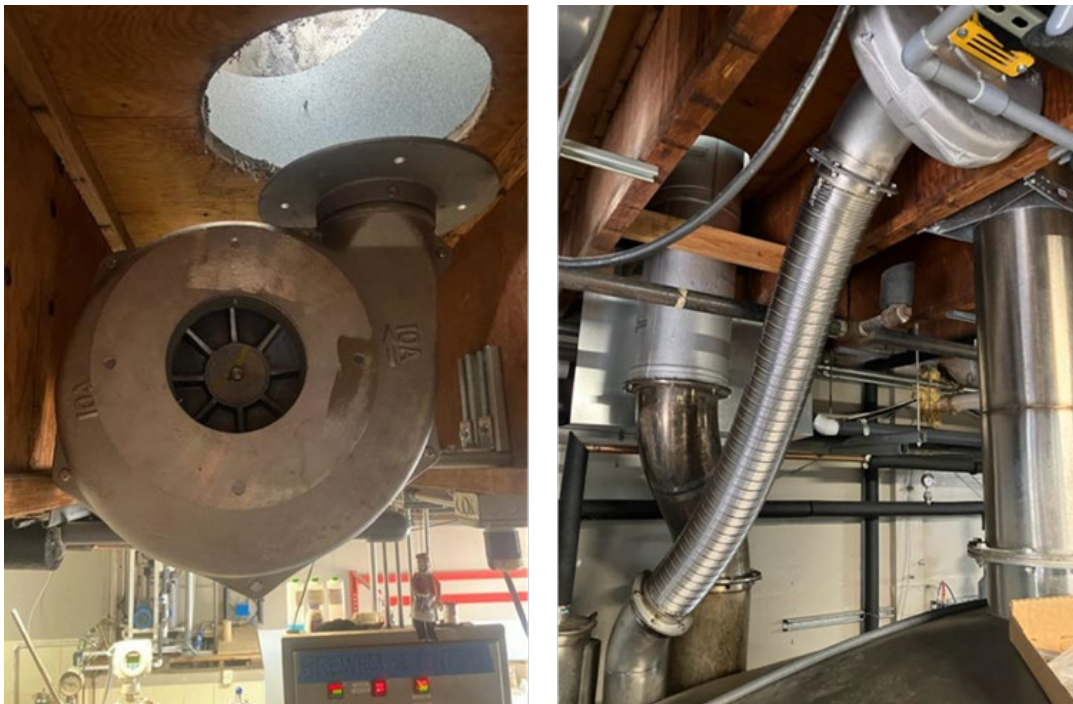
Figure 22: Draft Induction Fan Installation at Old Caz Brewery
