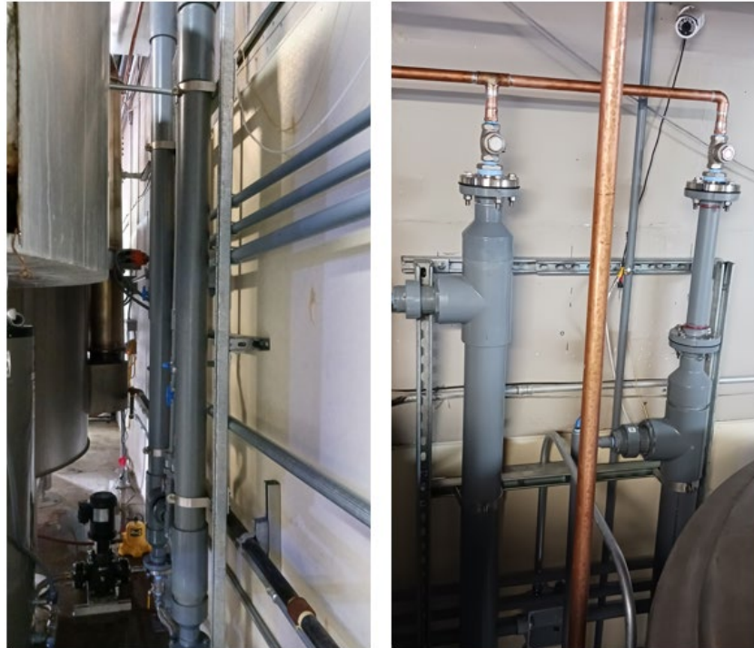
Figure 17: P-HEX Installation at Old Caz Brewery
