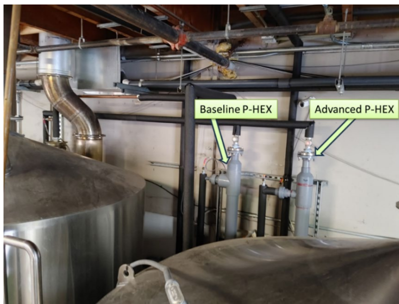
Figure 6: Baseline and Advanced P-HEX Installation at Old Caz Brewery
